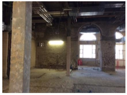
In addition to the brick arches there is a mezzanine floor which serviced plant, once the services are disconnected we propose to demolish the slab using a Brokk (demolition robot). This method will limit the vibration on the existing building.
