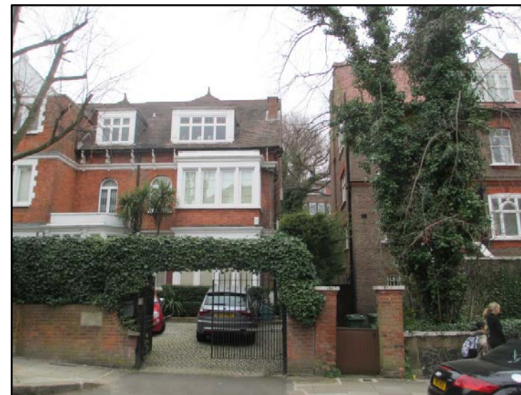
Photo 3: No 28 Netherhall Gardens
