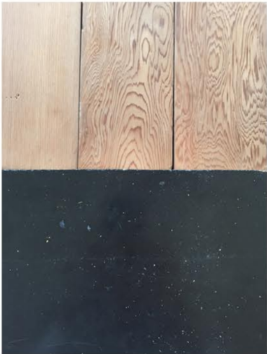
polished concrete floor throughout lower ground floor including proposed extension with reclaimed dougls fir timber panelling internal walls of the extension
