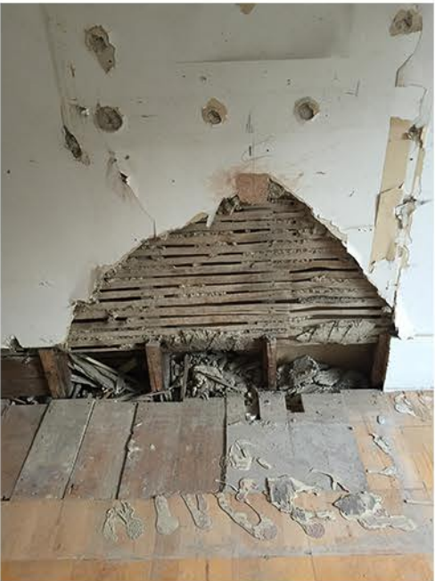
First floor original part timber floor, lathe & plaster and original part cornice
