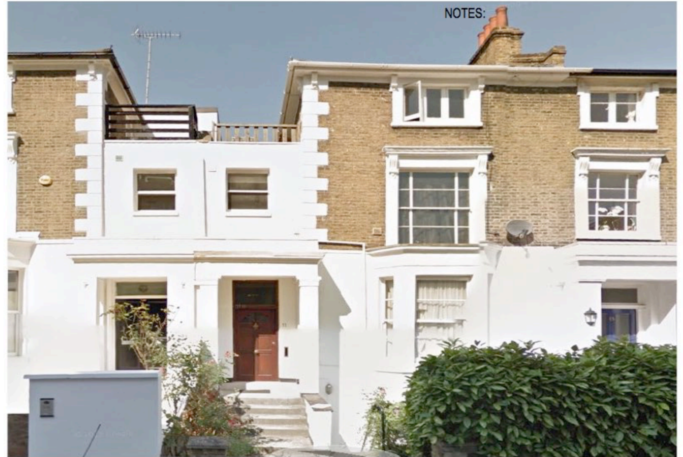
1. Front view from Greville Road
