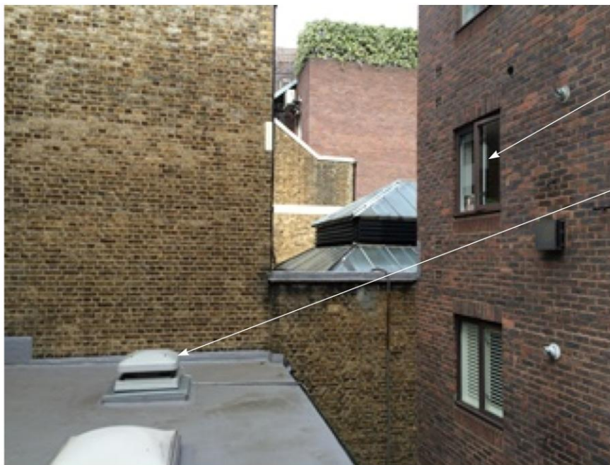
Residents windows overlooking flat roof.
