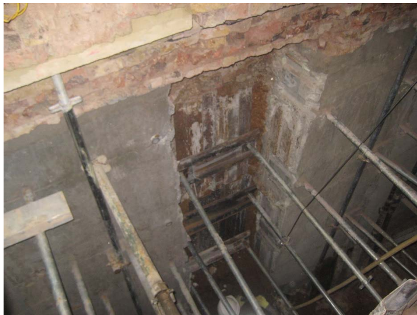
Figure 6 Example of trench sheet back propping
