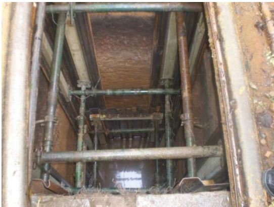
Figure 3 Propping examples
