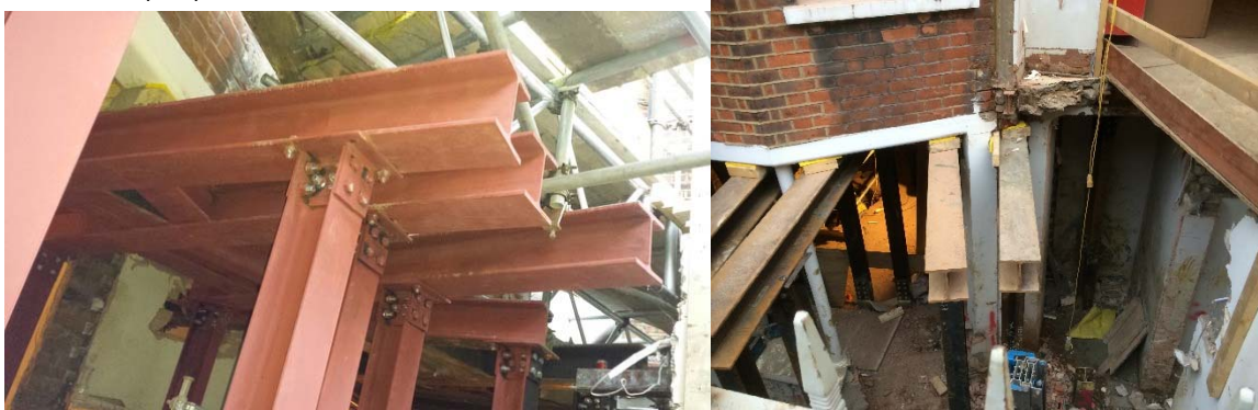
Figure 1 Example of needling to existing wall
