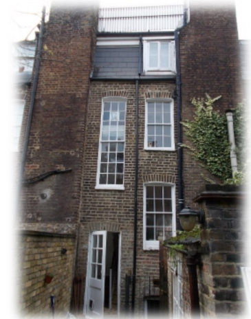
A view from the rear of the property
