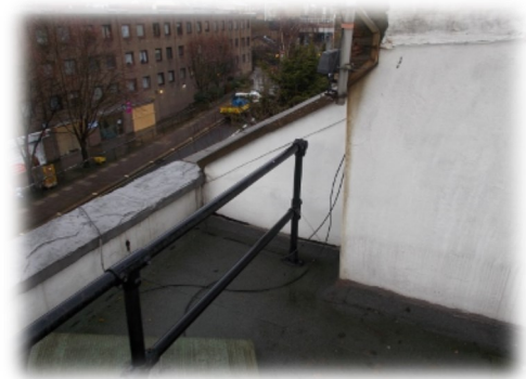
The existing railings situated to the front
