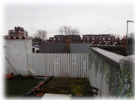
The rear edge of the existing terrace
