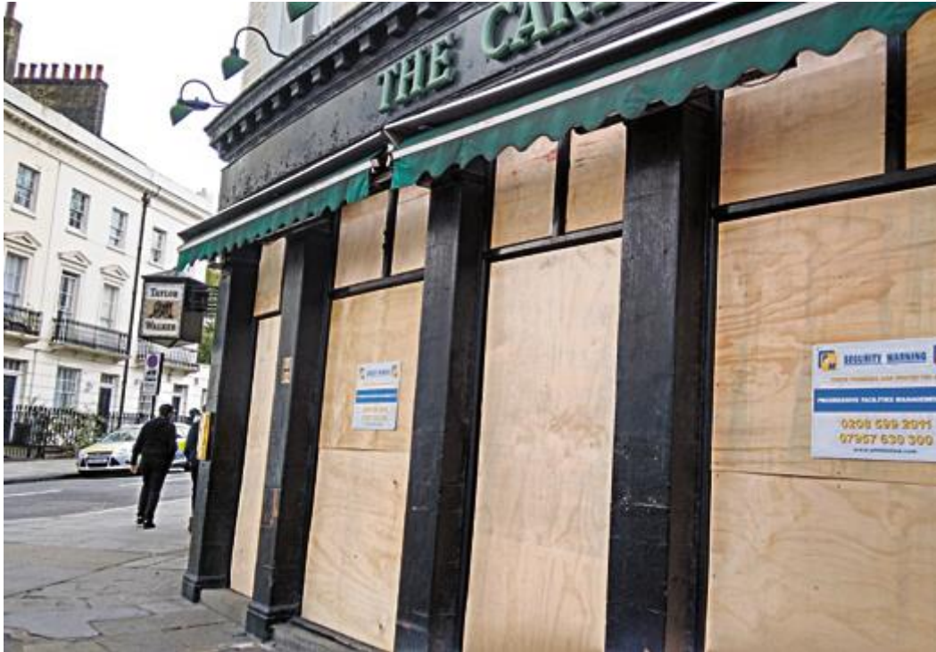
Boarded-up Carpenters Arms in King's Cross
