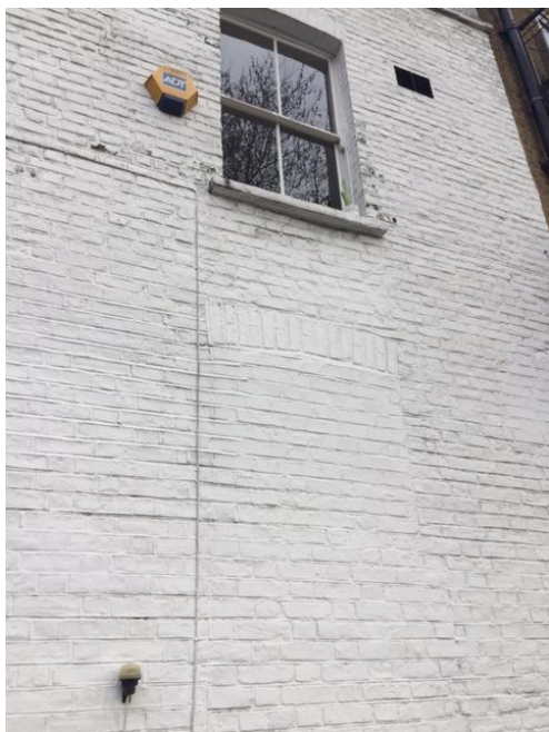
Photo 12 (above): Close-up of ground floor bricked up window to be re-instated on southern elevation of 49 Highgate High Street
