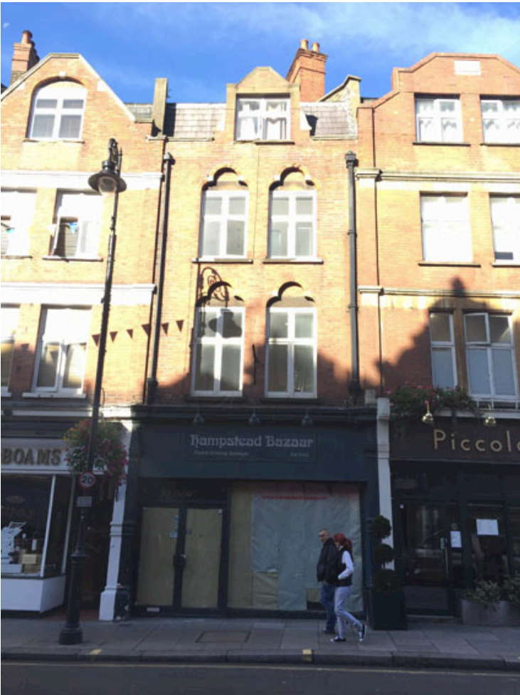
Photo of Existing Full Elevation
