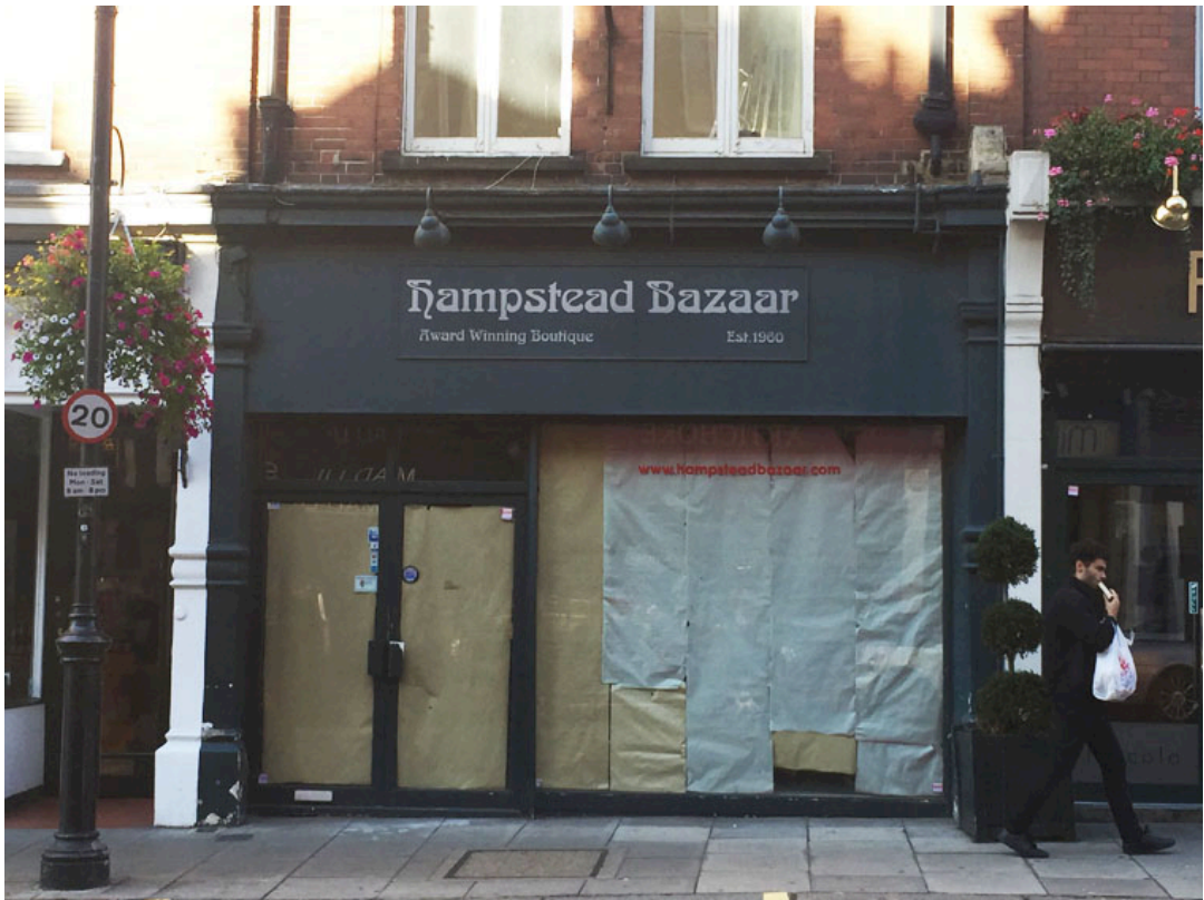
Photo of Existing Shopfront Elevation
