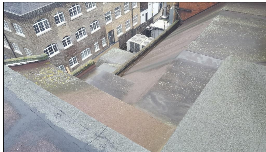
Photo 9: Examples of sloping felt roofs on B1.
