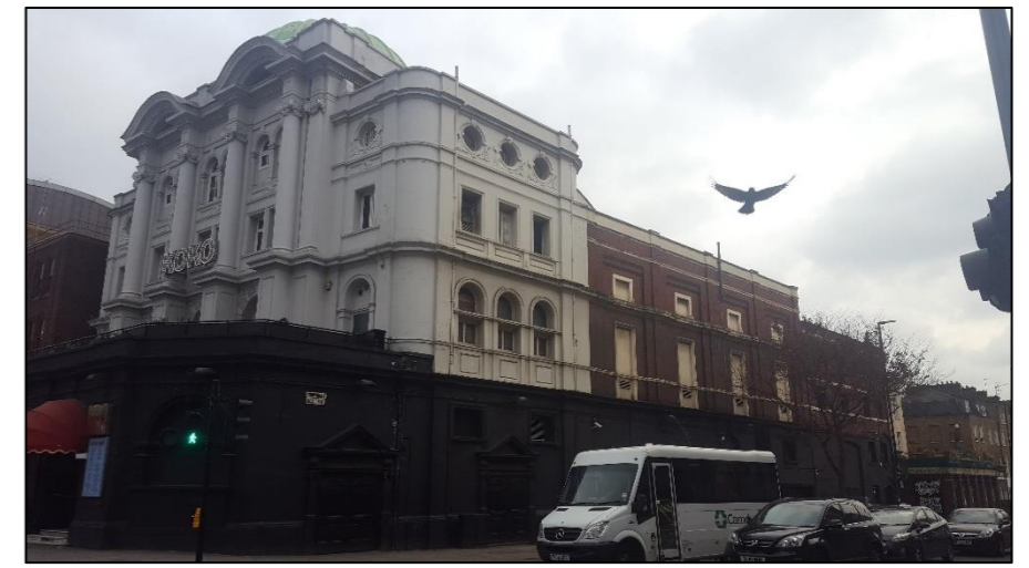
Photo 2: Looking north-east at B1.
