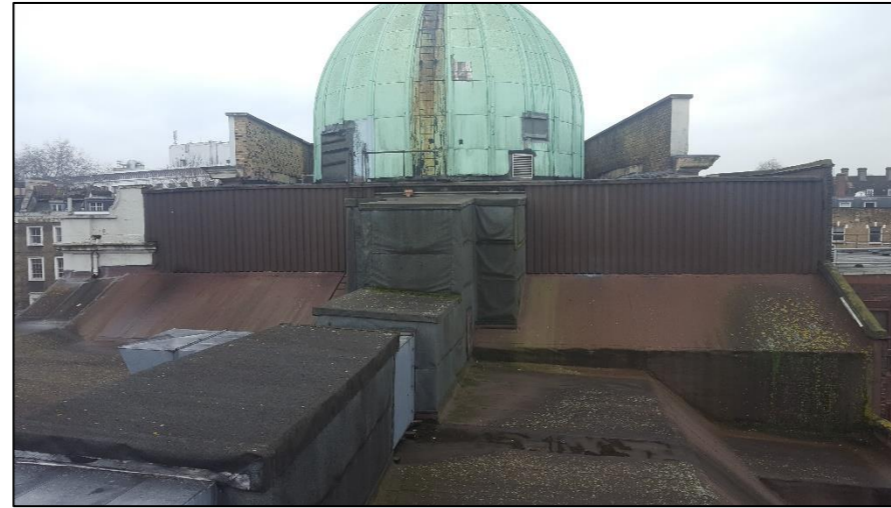
Photo 7: Looking west at the dome from the roof of B1.
