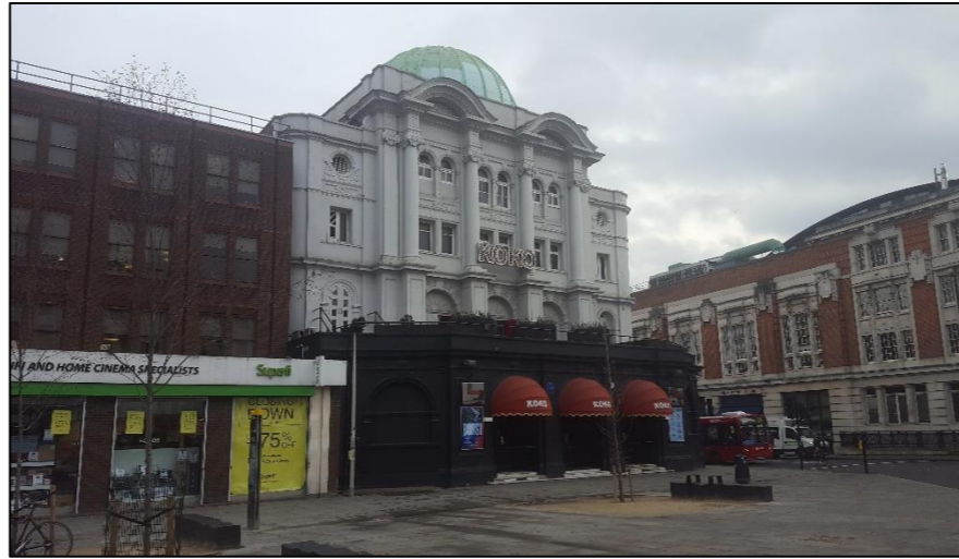
Photo 1: Looking south-east at the front (western end) of B1.
