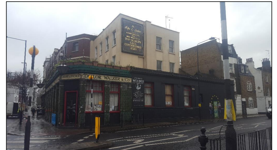
Photo 4: Looking west at the rear of B1.
