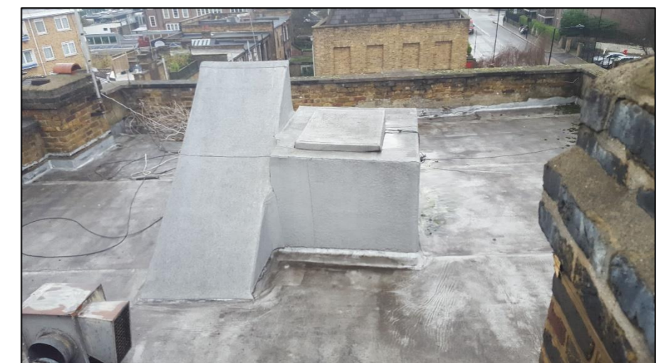
Photo 12: The roof of the public house section of B1.
