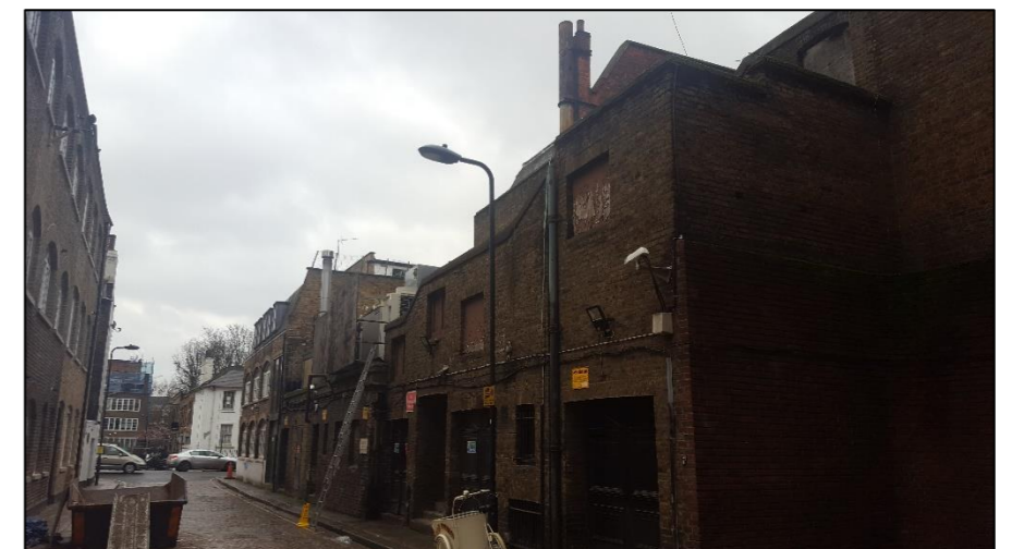
Photo 6: Looking east along the northern elevation of B1.
