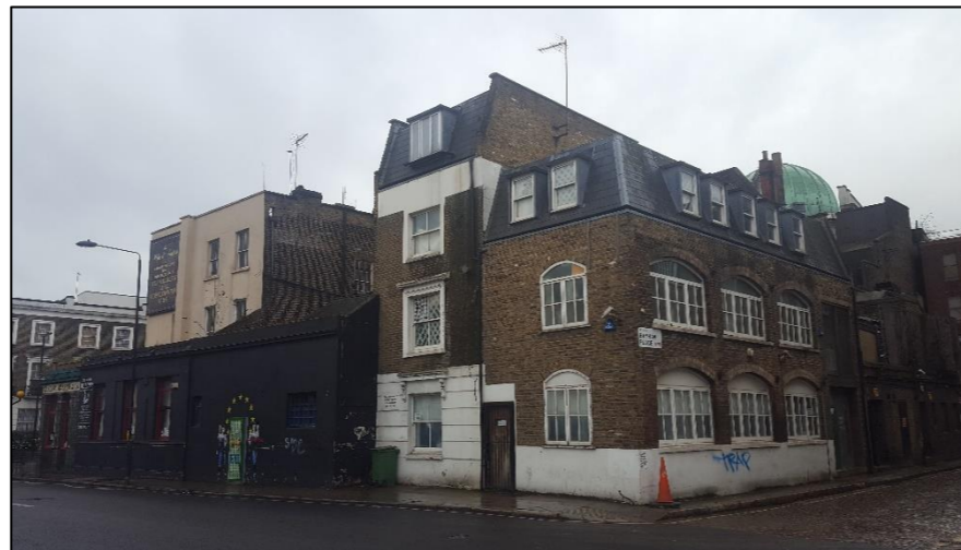
Photo 5: Looking south-west at the rear of B1.
