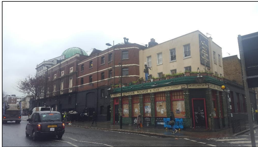
Photo 3: Looking north-west at B1.
