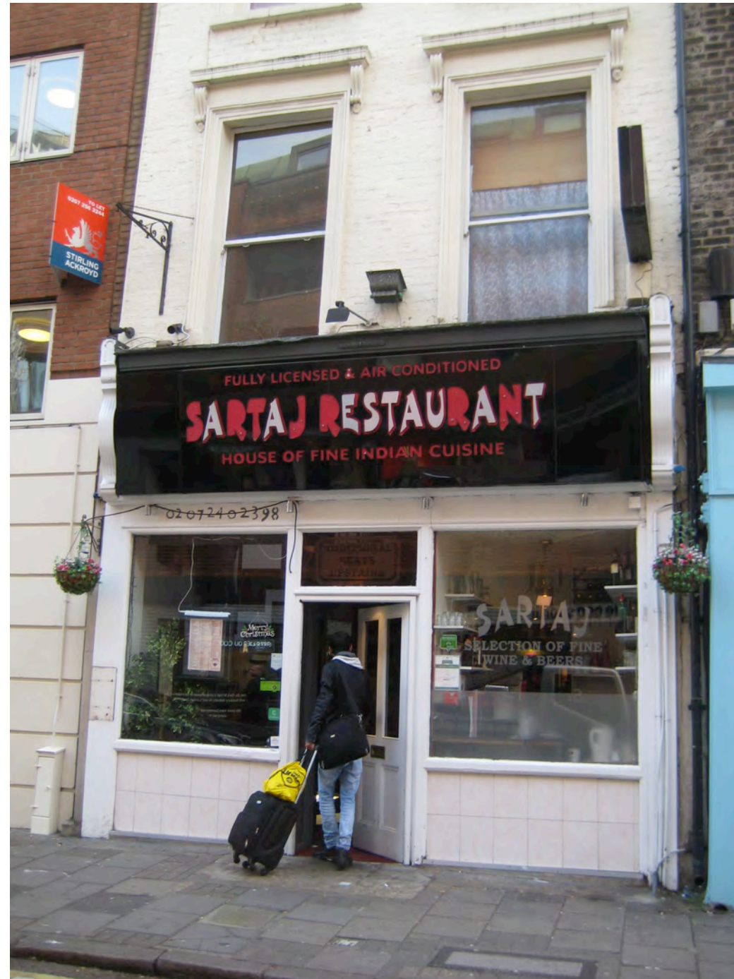
Photo of Earlam Street existing shopfront and signage
