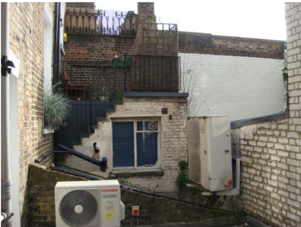
REAR 65 REGENTS PARK ROAD LOOKING WEST
