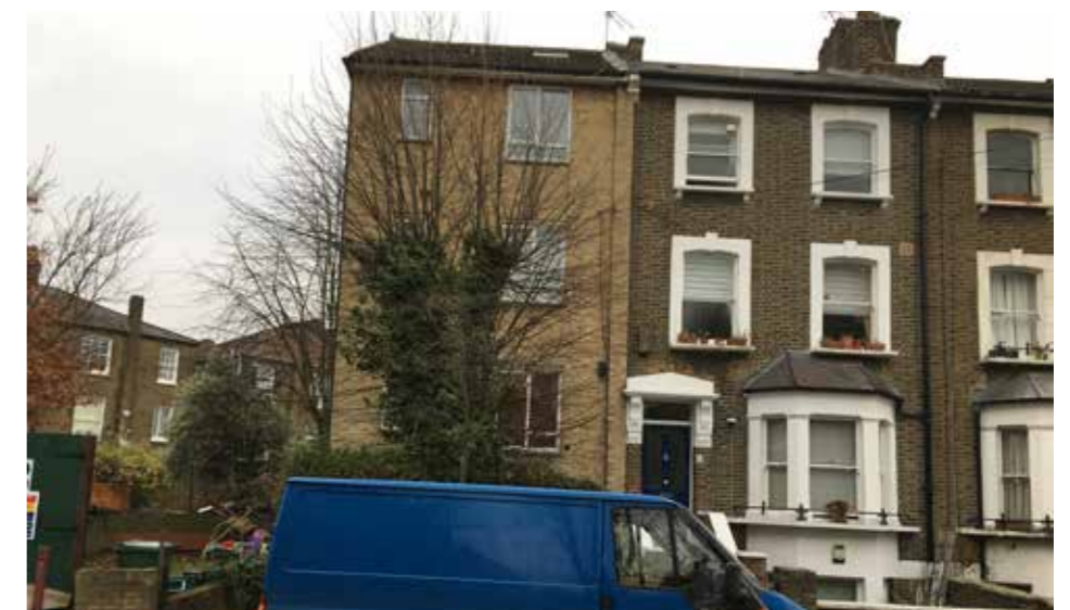
The Poplars Montpellier Grove
