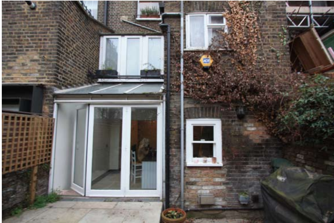
Showing relationship with neighbouring buildings
