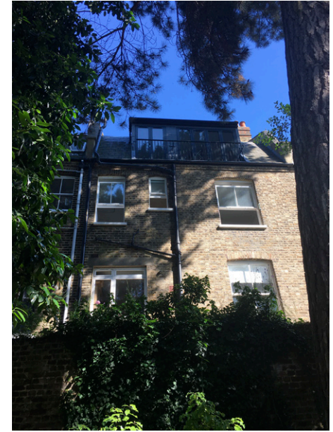
Rear view of rear of 12 Bisham Gardens
