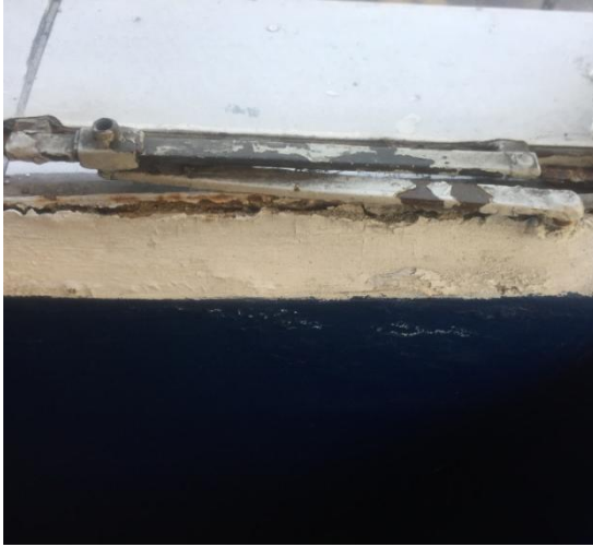
Examples of the extent of rust and damage
