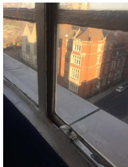
Examples of windows that do not close, undermining the existing use of the building
