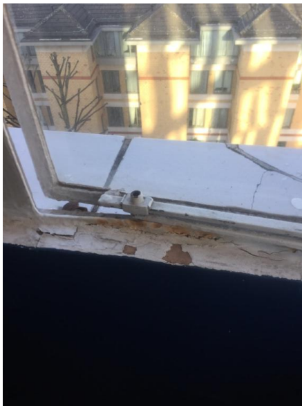
Examples of windows that do not close, undermining the existing use of the building
