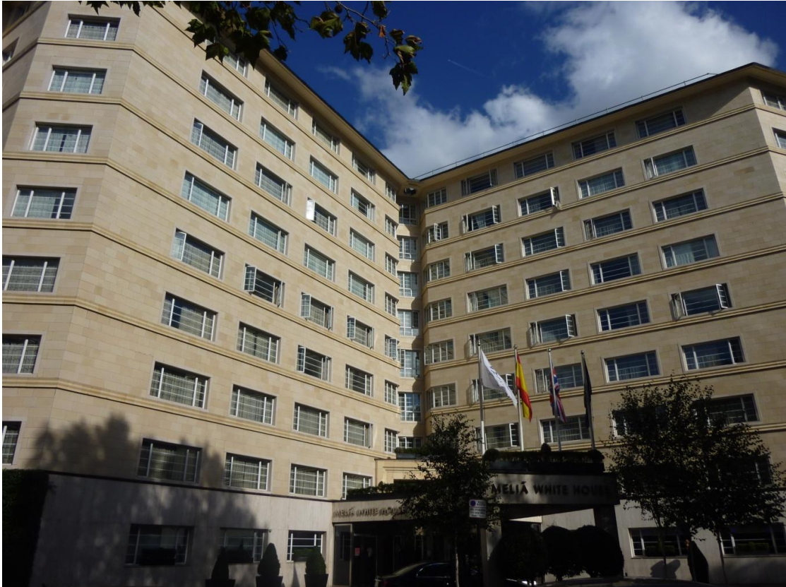
Main entrance on Osnaburgh Terrace, where all the original windows have been replaced.
