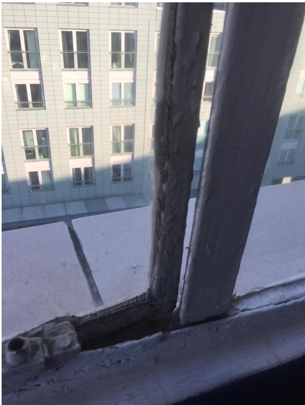
**Window Sample 07** – Rotten frame / warped frame / not possible to close – Not repairable
