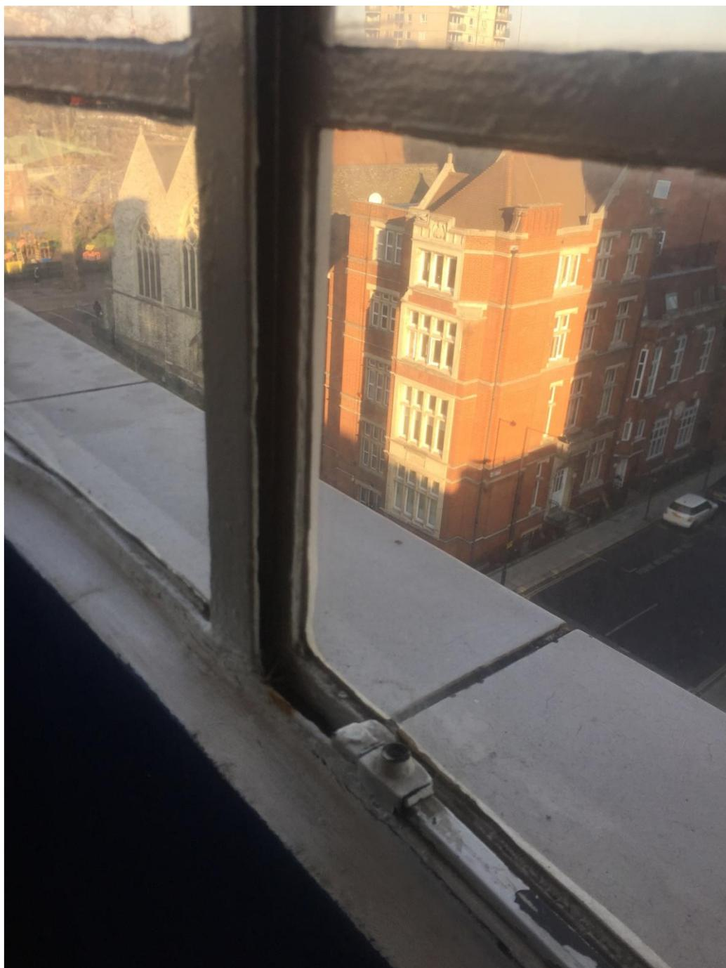
**Window Sample 06** – Rotten frame / warped frame / not possible to close – Not repairable
