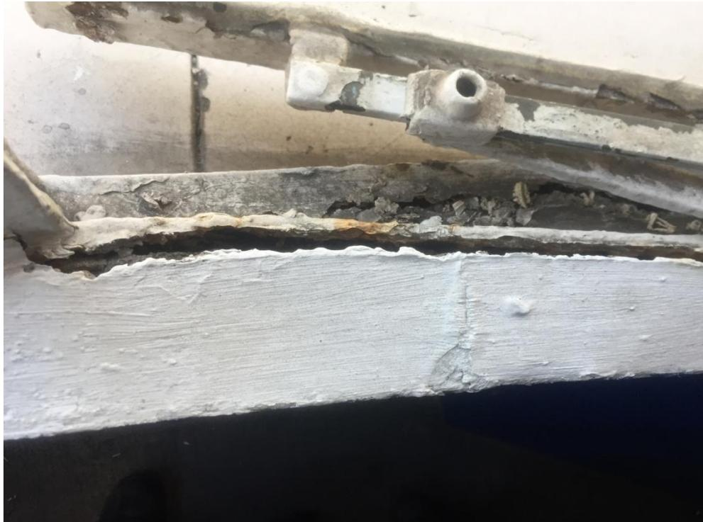
**Window Sample 03** – Frame corroded away from frame / not possible to close – Not repairable
