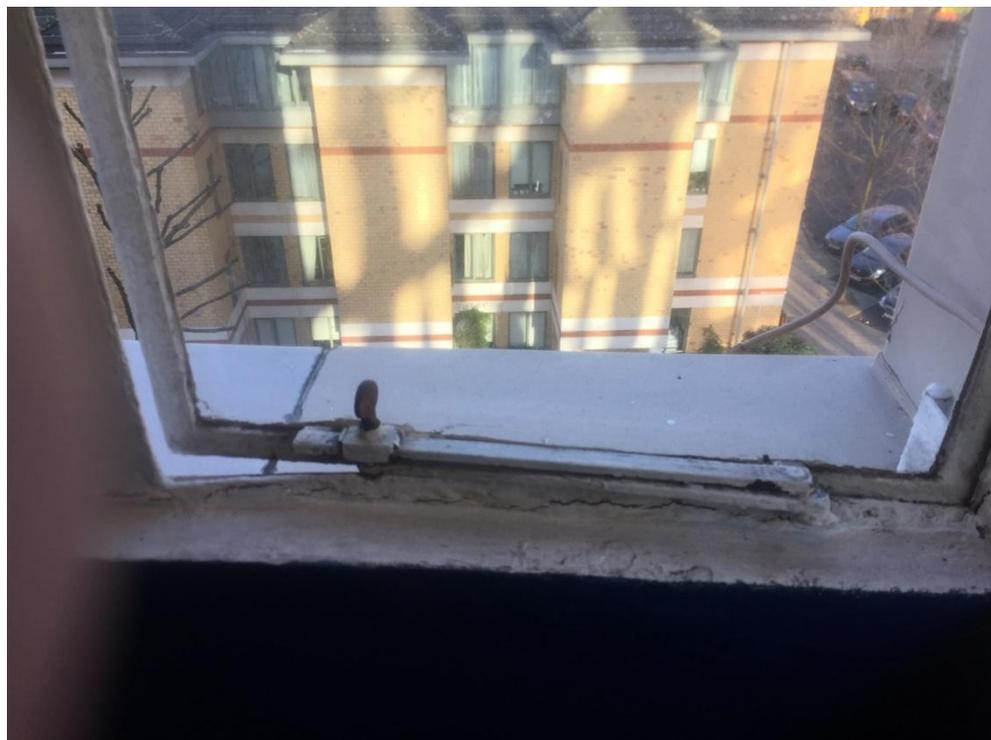
**Window Sample 04** – Warped frame / not possible to close – Not repairable
