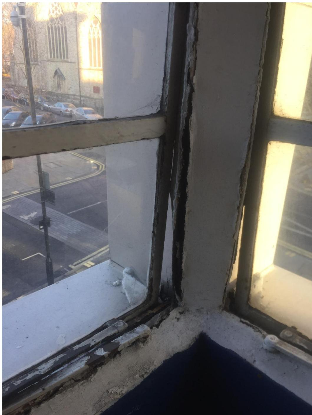
**Window Sample 08** – Rotten frame / warped frame / not possible to close – Not repairable
