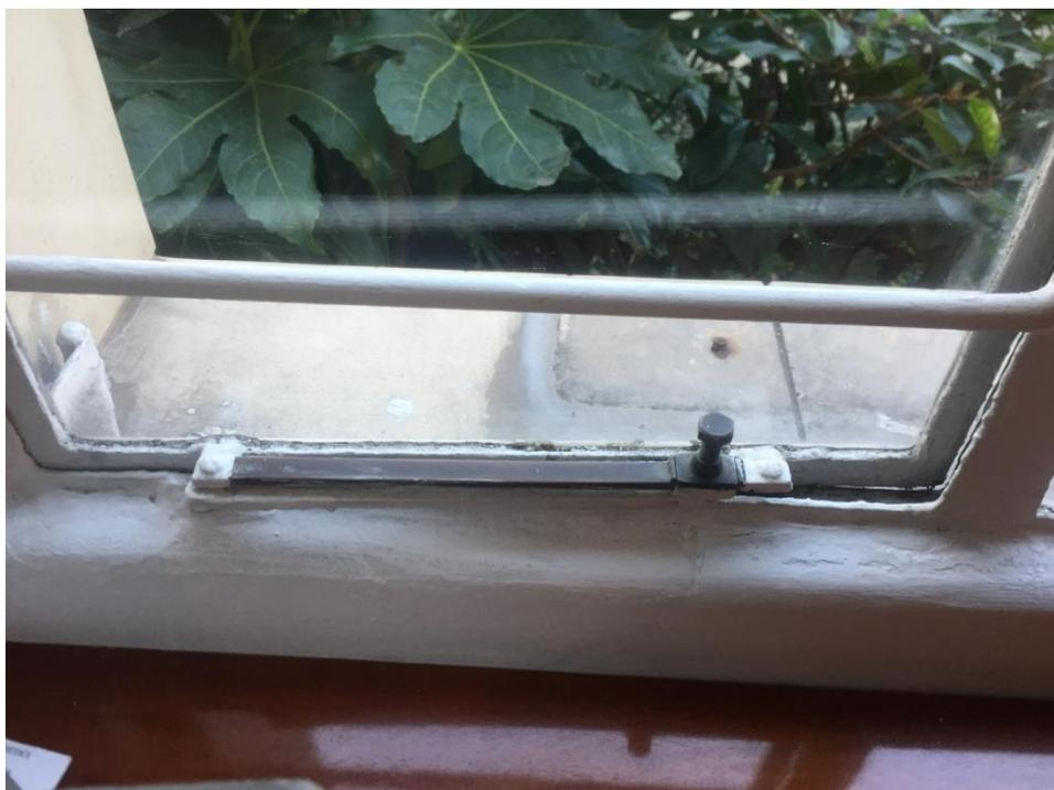
**Window Sample 02** – Frame rotten / warped frame / not possible to close – Not repairable
