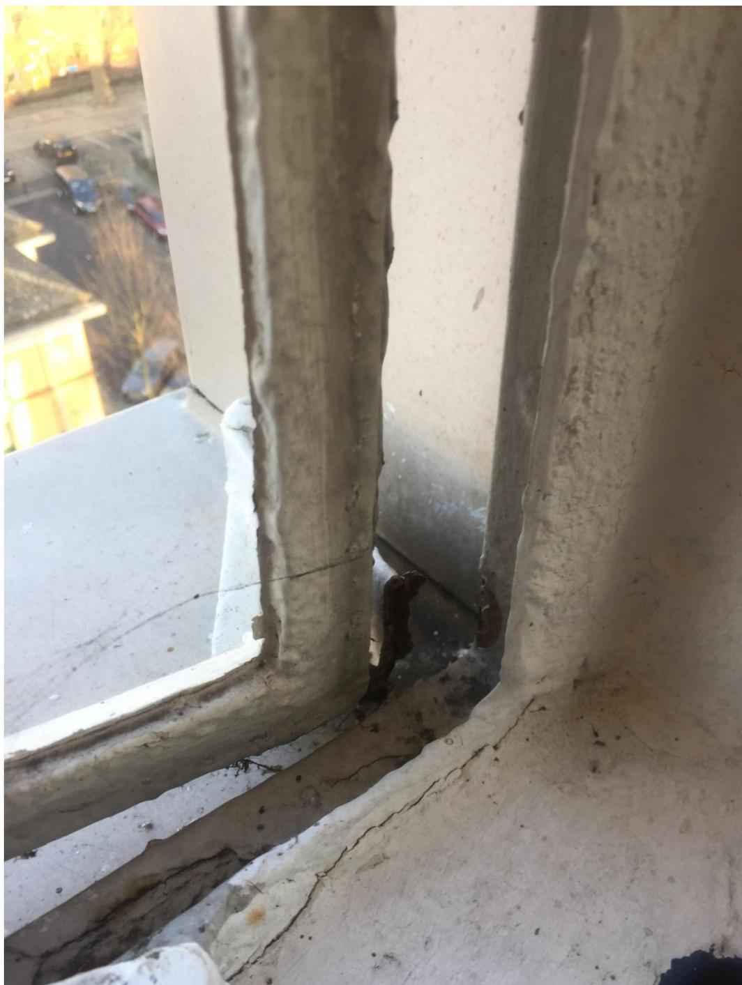
**Window Sample 05** – Rotten frame / corrosion of hinges / not possible to close – Not repairable
