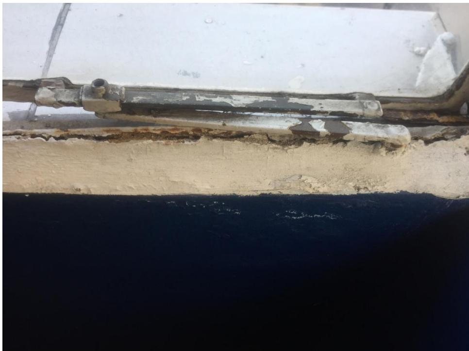
**Window Sample 01** - Frame rotten / closing mechanism broken – Not repairable
