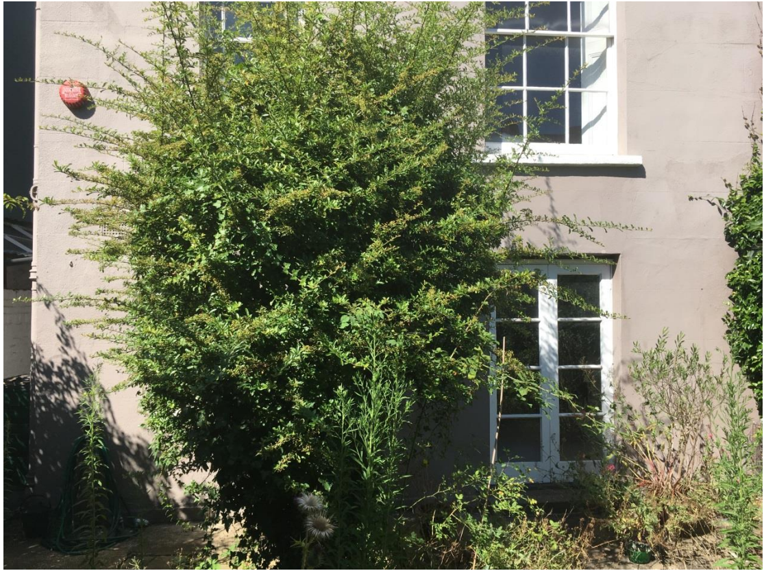
Picture 2 – Lower Ground Floor Rear Elevation
