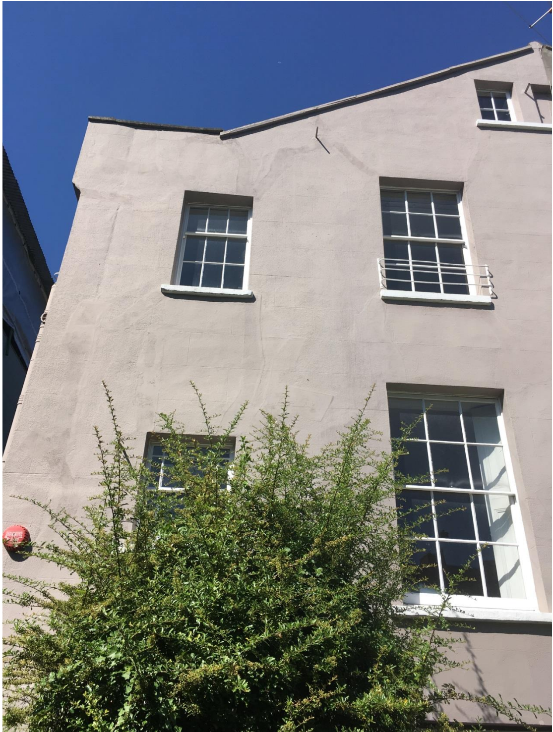
Picture 1 – Upper Rear Elevation
