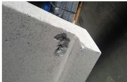
4: Spalled area exposing reinforcement.
