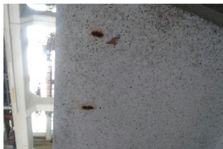
2: Visible corrosion staining, reinforcement too close.
