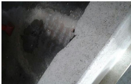
3: Breaks to faces of lead edge of stair tread.
