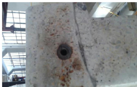
1: Visible corrosion staining and ferrous fixing.
