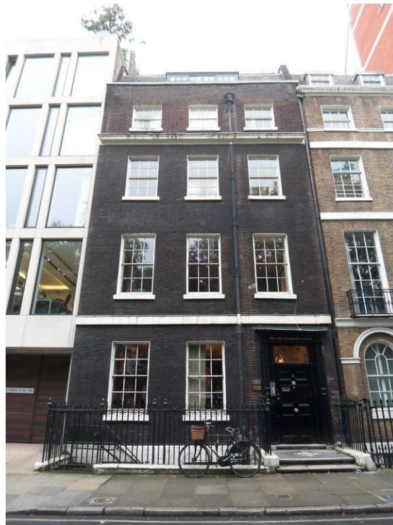
The Art Workers' Guild building at 6 Queen Square
