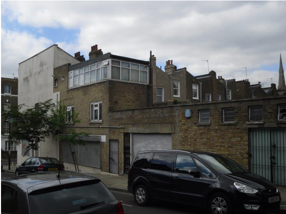
View – Rear of building (Montpelier Grove)
