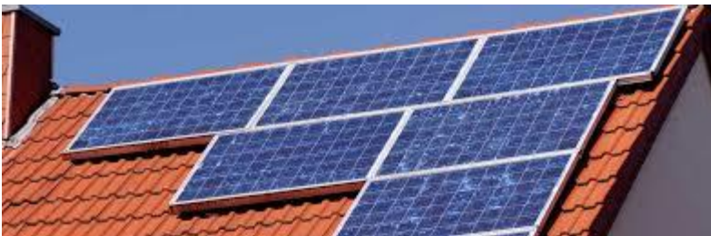
Figure 2: Typical PV installation to pitched roof
