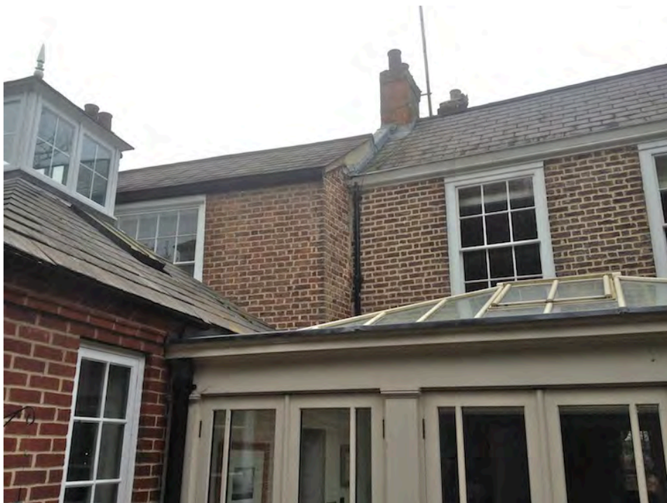
Rear [east] elevation detail, junction behind of the original house with old extension
