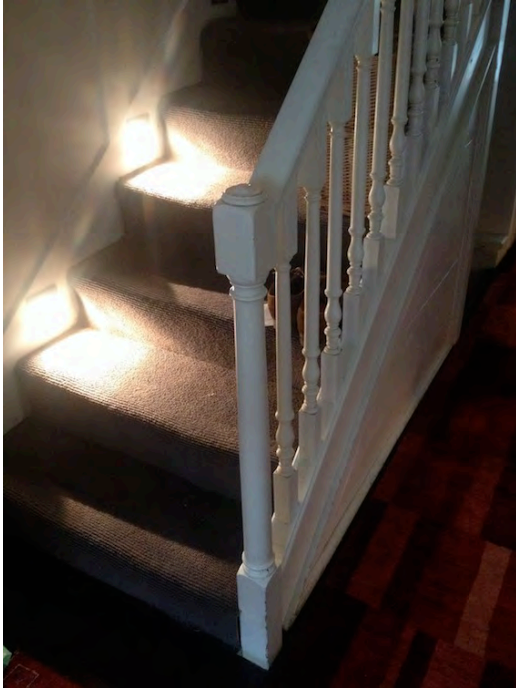
Detail at base of stairs
