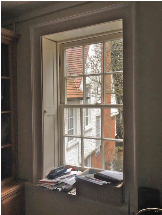
Detail of front window at first floor
