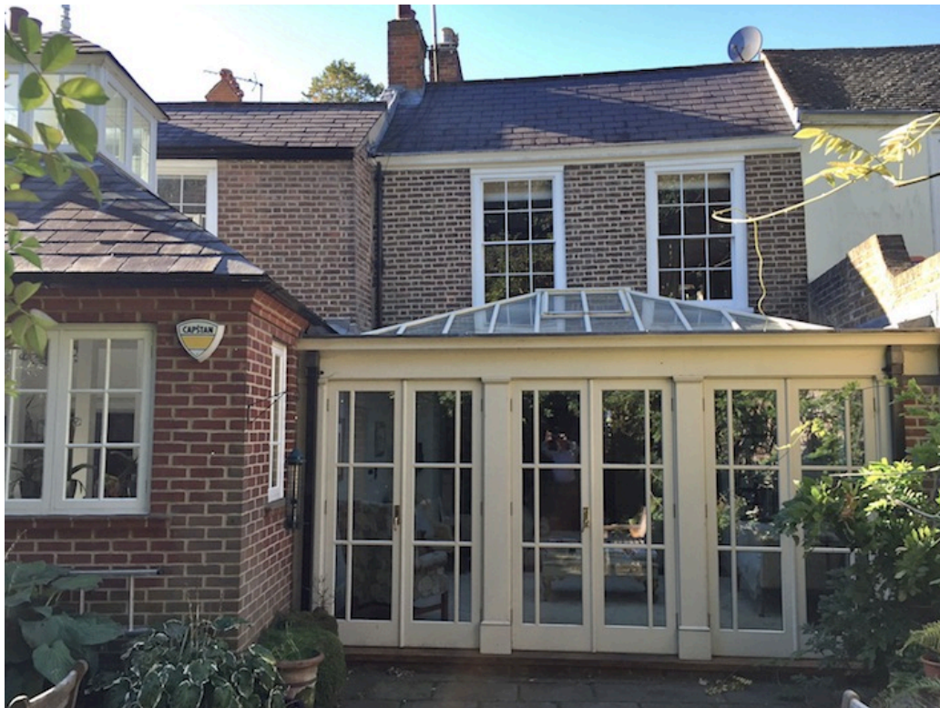
01 - View of the existing rear extension conservatory
