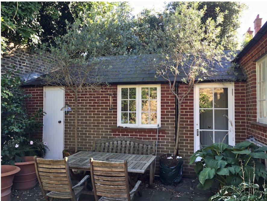
03 - View of the existing rear extension utility area
