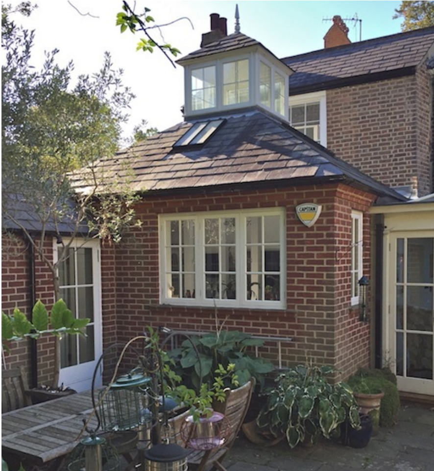
02 - View of the existing rear kitchen extension
