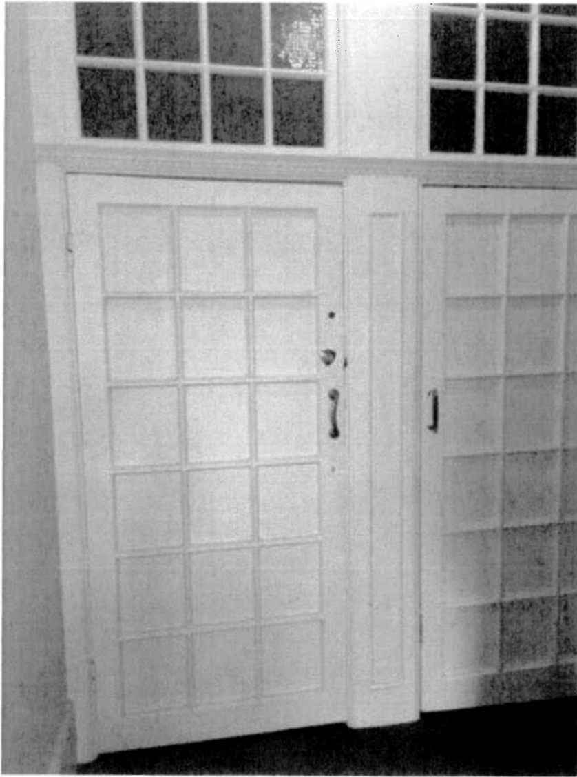
Access to the upper floors is provided to the left, with access to the ground floor flat provided to the right
