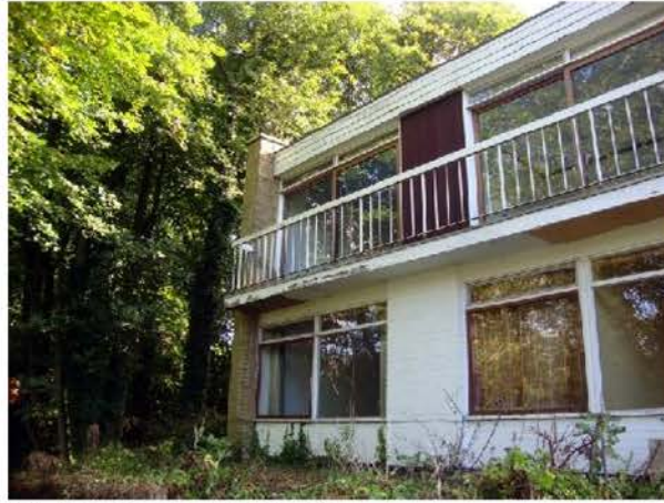
01- Existing property (rear)
