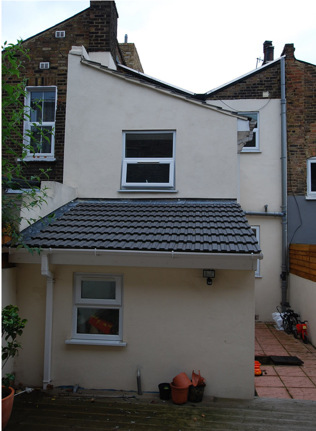
Rear facade from garden
