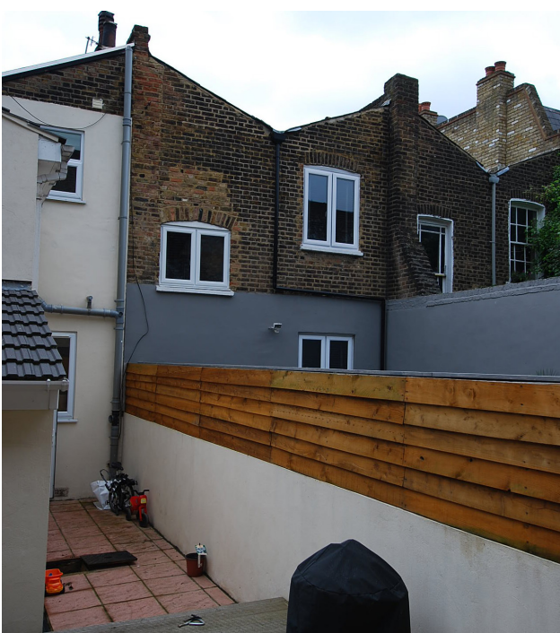
Party Wall with 4 Hadley Street
