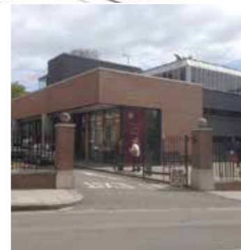
Gate 6: vehicular entry gates open from 6.30am -10.30pm. Manual operation
