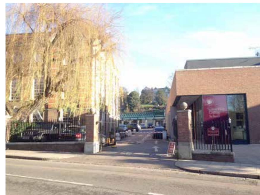
Entrance: View from Froggnal pavement
