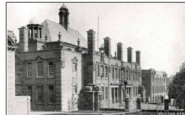
Early photograph showing an enclosed Froggnal Entrance
