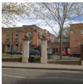
Gate 3: pedestrian entry - electronically activated: opens at 7.30am -8.50am, and 3.55pm (Monday - Thursday) On Friday 3.25pm to 4.30pm.Key pad exit system.
