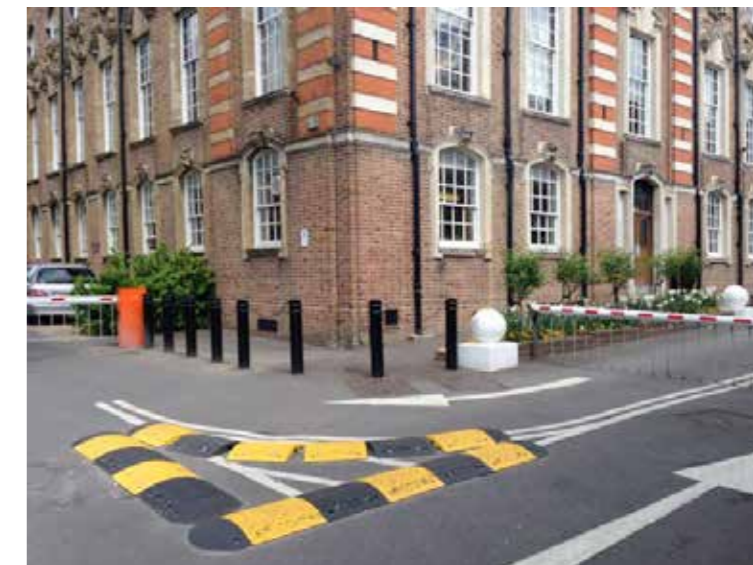
Entrance: View from within the School showing existing street furniture to the edge of the Listed Building
