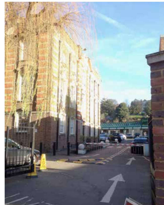
Entrance: View from boundary showing existing Vehicular Entrance
