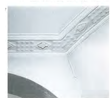
Typical cornice of period 1800-1830. The motifs are derived from classical elements. From Charles Dickens House.
