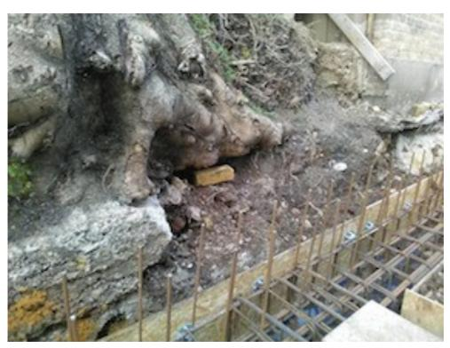
3.5 Photograph of lateral roots to west with void beneath tree root plate to west and ad hoc cast concrete infill combined with loose topsoil
