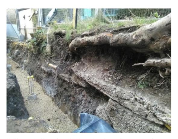
3.5 Photograph of base of tree / initial root plate where wall and associated foundations have been removed with new ground beam cast. Note void beneath tree to east also and abrupt deflection of tree root upon the concrete infill
