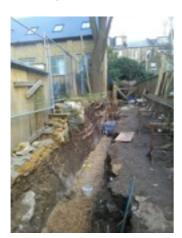
3.2 Exposed base of tree T1 further to full removal of wall dismantling of previous foundations and casting of ground beam atop pile foundations as viewed in an westerly direction
