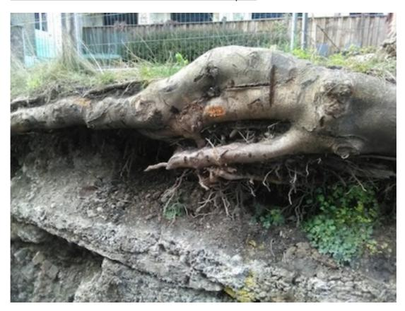
3.7 Photograph of base of tree / initial root plate where wall and associated foundations have been removed with new ground beam cast. Note void beneath tree to west also and abrupt deflection of tree root upon the informal concrete infill which exists directly beneath the tree
