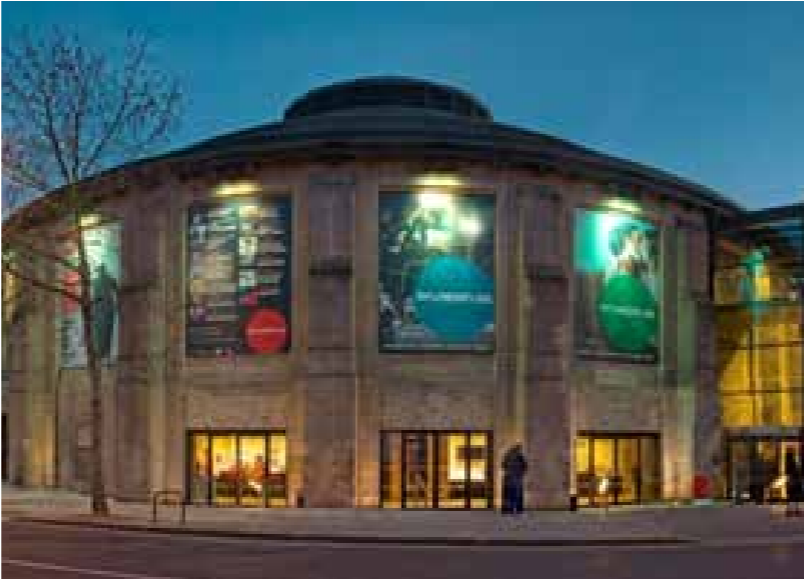
The Roundhouse Refurbishment
