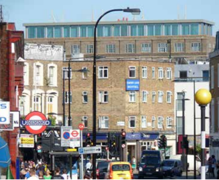
Belmont Street warehouse conversion and roof extension
