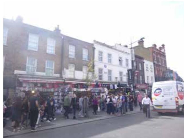
View of units 253-259
