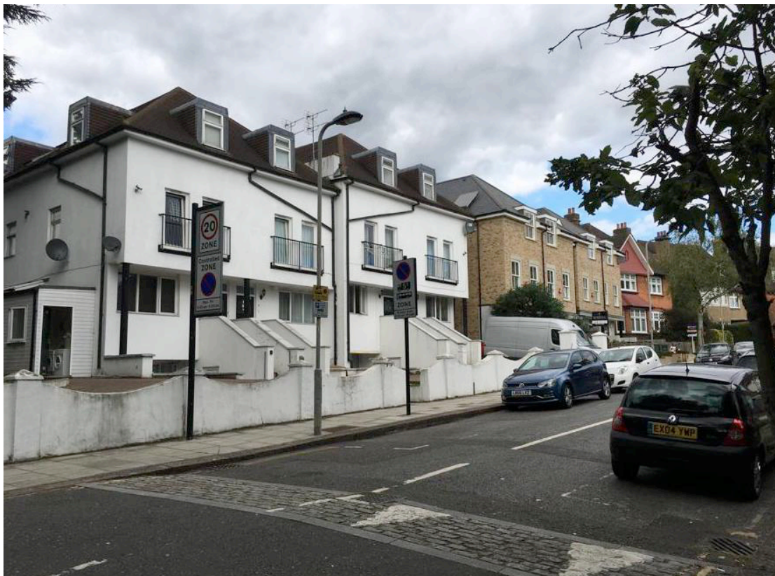
Front and west facade in the context viewed from corner Shootup Hill / Kingscroft Road
