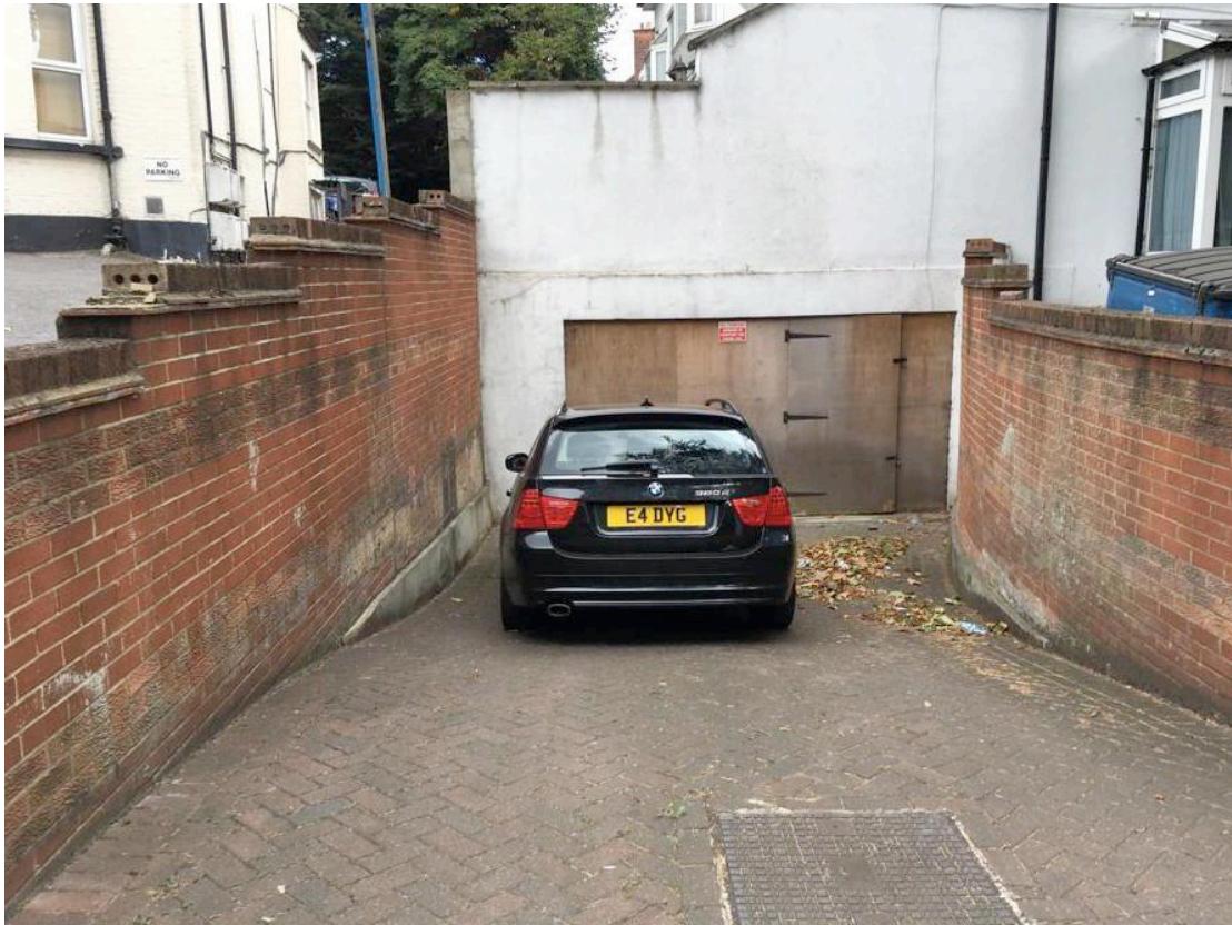
Unightly side garage entrance blocked off
