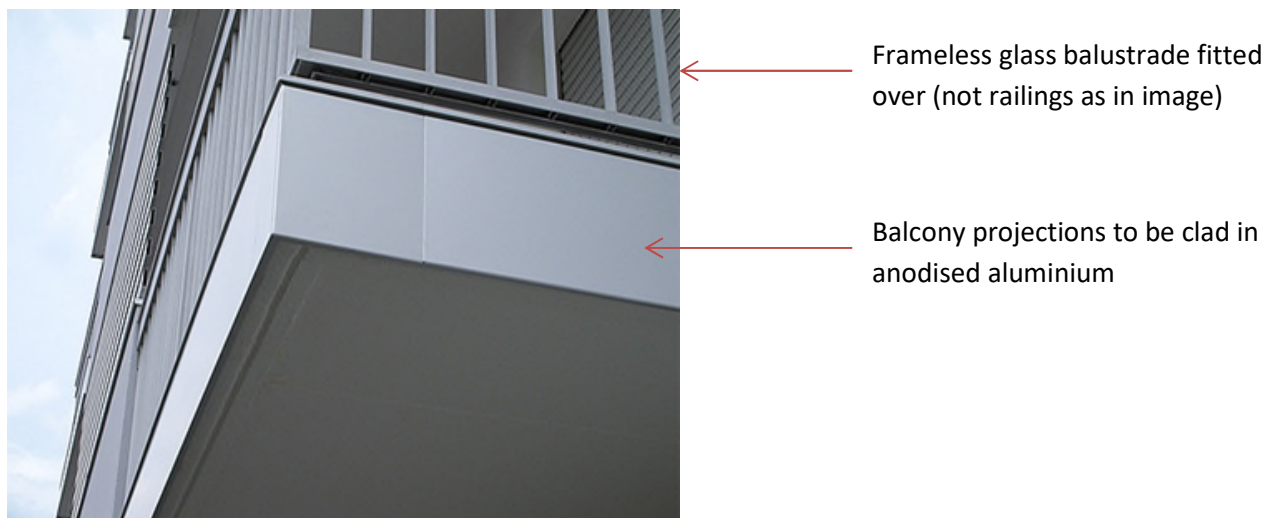
Proposed aluminium cover panels to balcony projections
