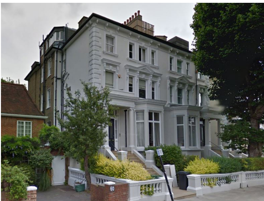
Fig 2. 62 Belsize Park Gardens front facade
