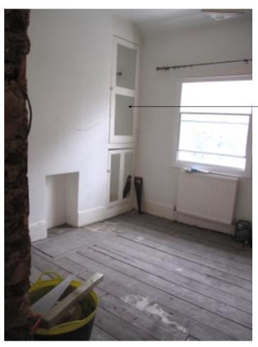
Non original mirrored glass glued to surface of cupboard. Very difficult to remove glass without damaging the wood panels behind.
