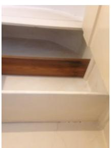
Non original slats and patching work has been carried out on the cupboard, which is unsightly and has caused cracking.
