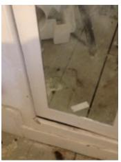
Warped doors and chips around door frame
