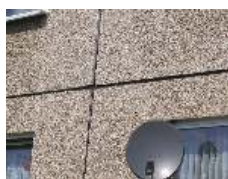
[Pic. 3]: Typical building structure with access to existing spaces
