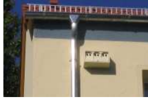
[Pic. 6]: Example of installed 1SP
