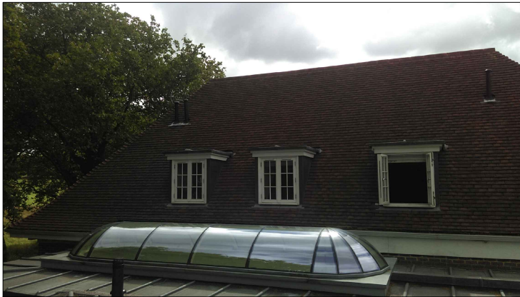
EXISTING ROOF LANTERN
