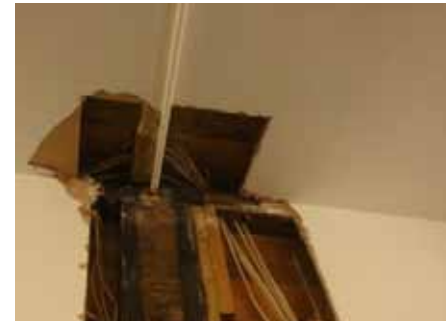
DT1: exposed middle post with steel support
