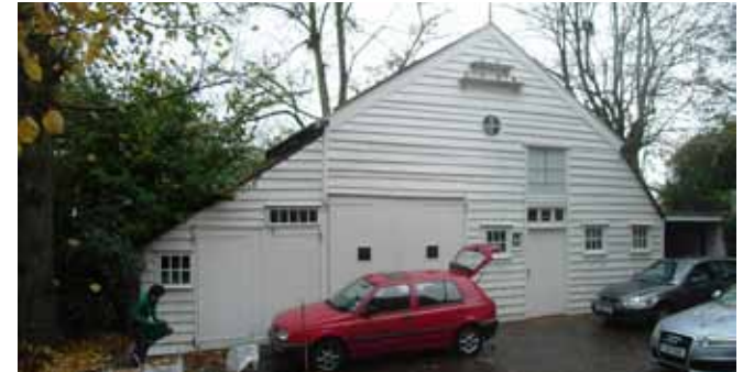
Existing front facade
