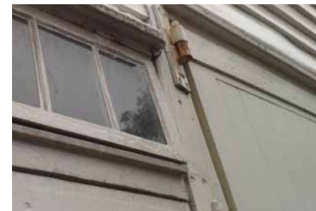
DT3: external wall gate post
