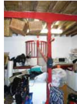
Ground floor right bay
