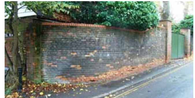
Existing condition of garden wall
