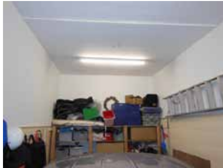
Ground floor centre bay
