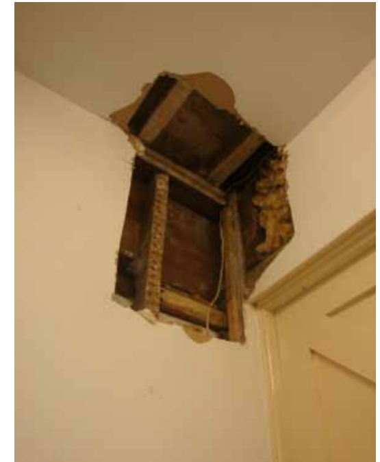
DT2: exposed external wall post
