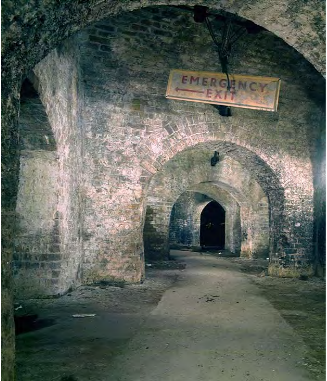
Camden. The Camden Catacombs , as they have become known are were once owned by British Railways but have now passed into multiple ownership. Some sections were demolished during the redevelopment of the area while other sections belong to Camden Market who discourage access.
