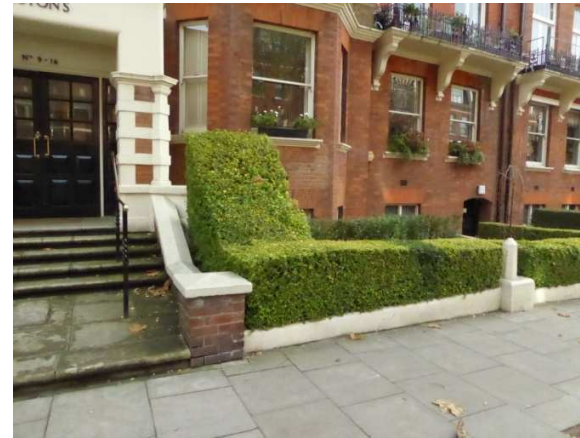
10) Older section of wall, evidently original, which has been reduced in height and rendered. Pier capped with painted stone obelisk.
