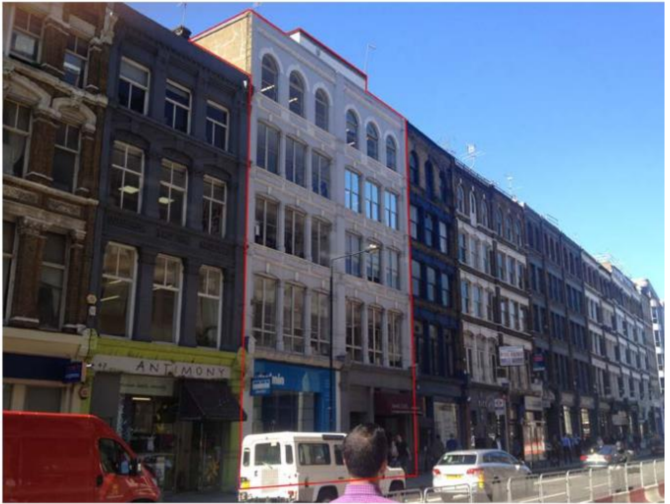
Photo 3 (above): Front elevation from Farringdon Road
