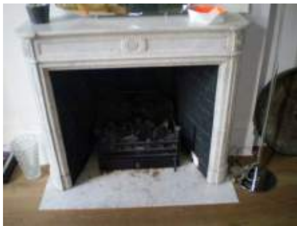
First floor front room. Non-original marble period mantelpiece and hearth with free-standing grate - No Significance. High architectural merit. Good quality and worthy of retention.
