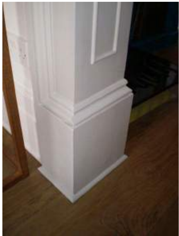
First floor front room. Detail non-original arch lining, architrave and plinth - No Significance. Low architectural merit.
