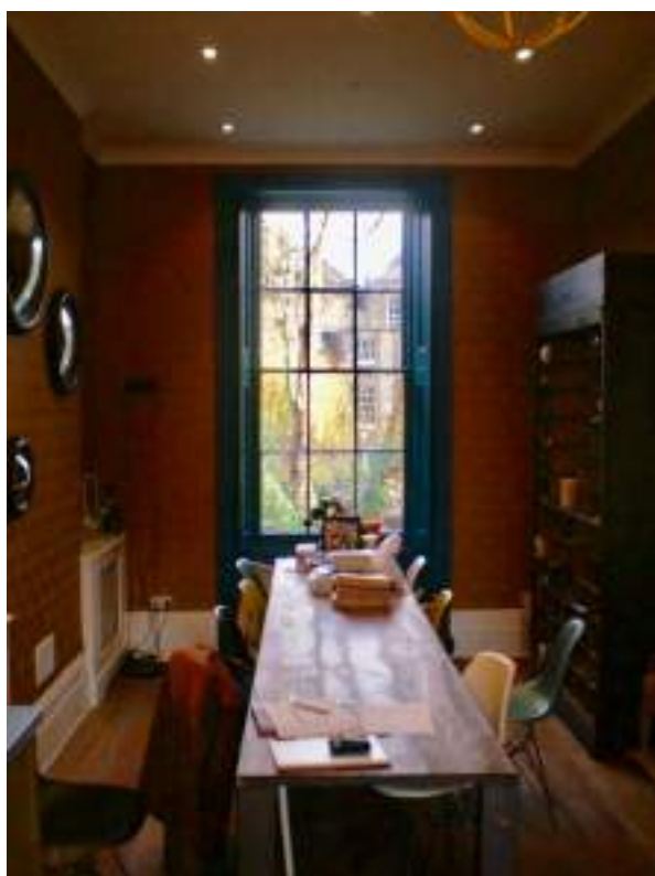
Ground floor rear room. Overall, High Significance. Original window shutters, panelling and architrave - High Significance.
