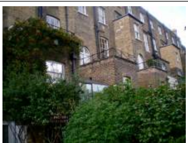
The rear of the houses to the north side. Taller brick rear extensions.
