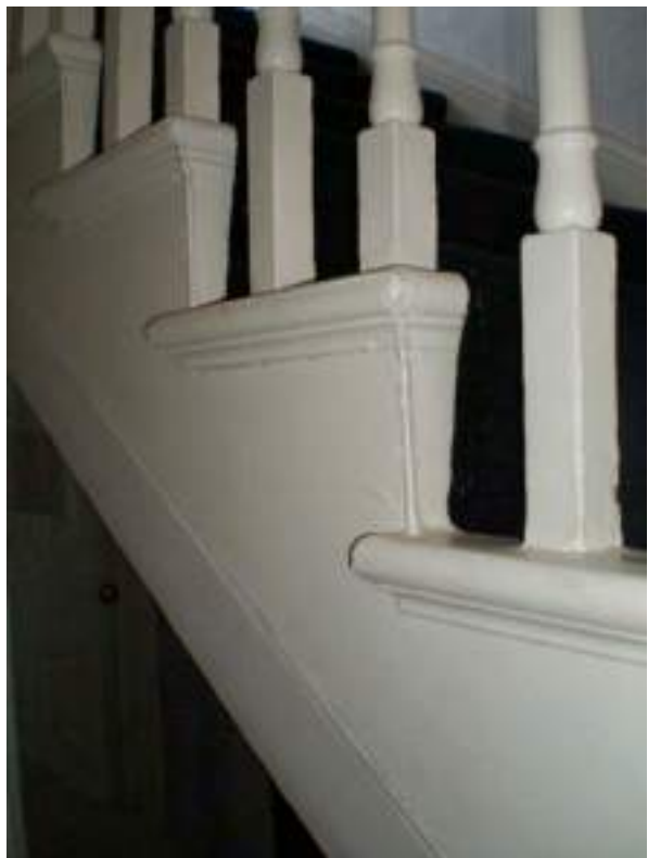
Open string staircase with bull-nosed treads and turned bannister rails. Original feature - High Significance.
