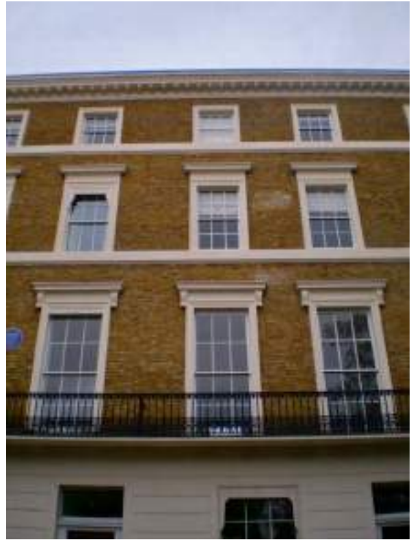
First floor stone balcony with cast iron railings. Windows with stucco architraves and corniced heads to first and second floors, Sliding sash windows - High Significance.
