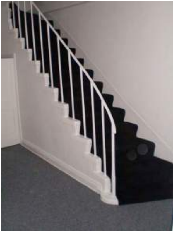
Basement stone stairs with cast iron railings - High Significance.
