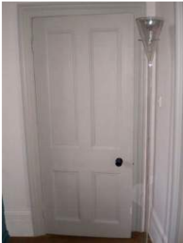
First floor rear room. Original four-panelled door - High Significance.
