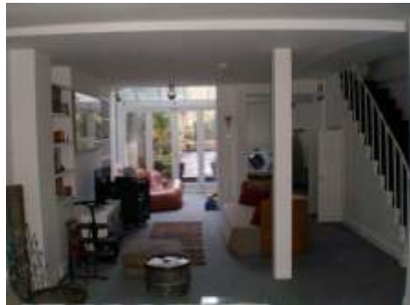
Basement Rear Room - Negligible Significance. All internal partition walls removed - harmful modern alterations.
