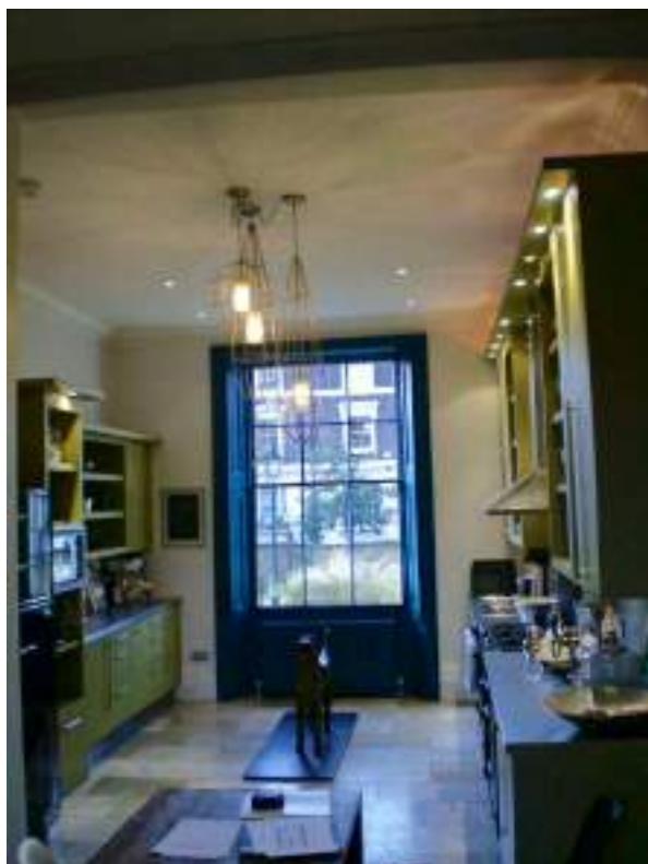
Ground floor front room. Overall - Medium Significance. Stone flooring - Harmful modern alteration.
