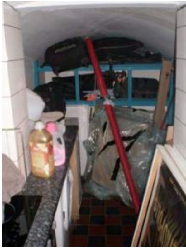
Vault under pavement. Low Significance.
