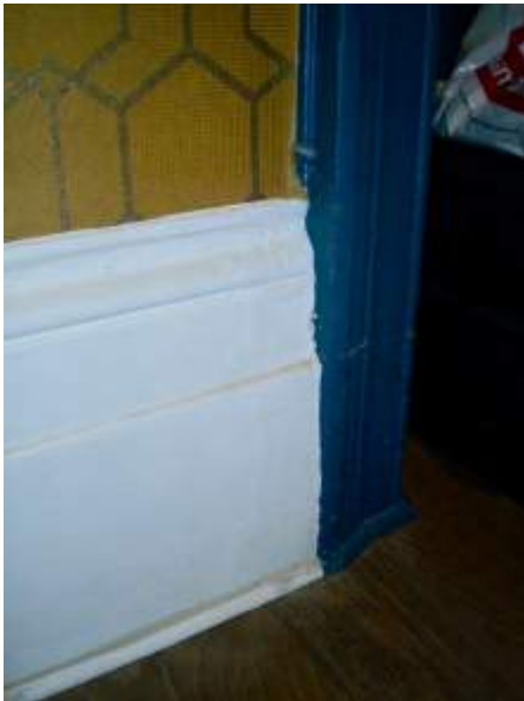
Ground floor rear room. Detail of original skirting board - High Significance.
