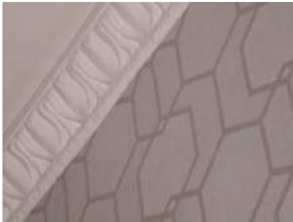
Interior of front door. Non-original overboarded and mouldings applied - Harmful modern alteration.
