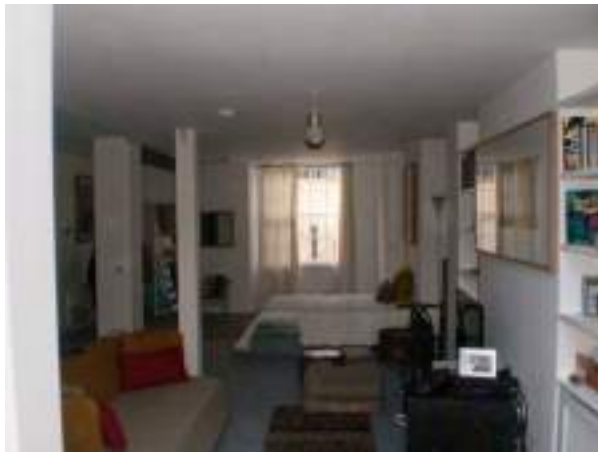
Basement Front Room - Negligible Significance. All internal partition walls removed - harmful modern alterations.
