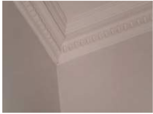
First floor rear room. Non-original period ceiling cornice - No Significance. Medium architectural merit. Good quality and worthy of retention.
