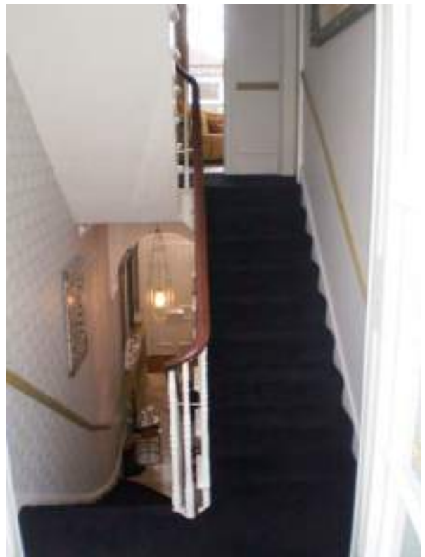
Second flight from half-landing to first floor. Original feature - High Significance.
