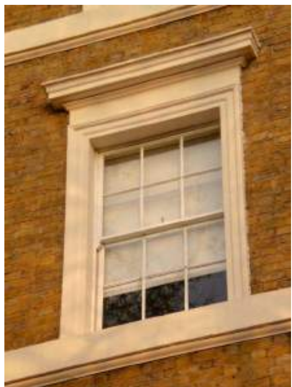
First floor stone balcony with cast iron railings. Windows with stucco architraves and corniced heads to first and second floors, Sliding sash windows - High Significance.
