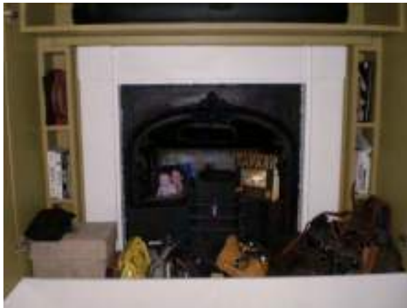
Second floor front room. Original fireplace mantelpiece and register grate hidden inside wardrobe- High Significance.
