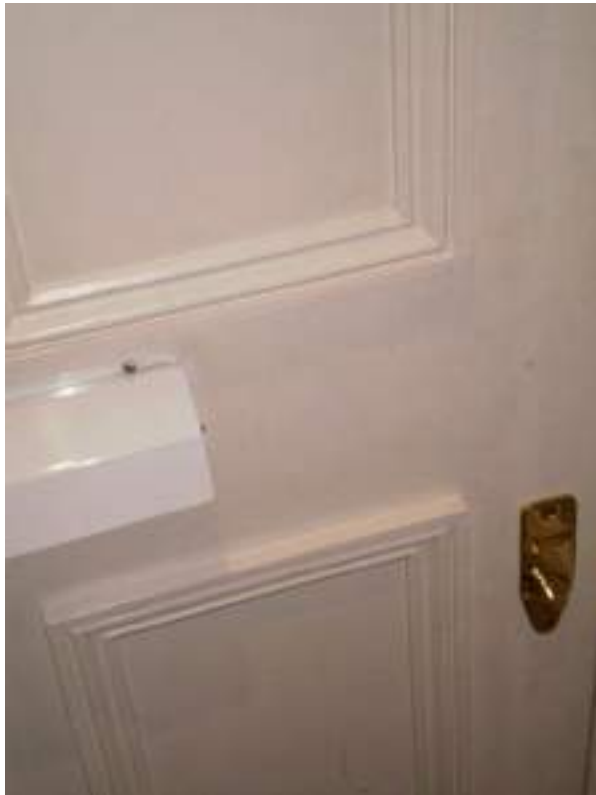
Interior of front door. Non-original overboarded and mouldings applied - Harmful modern alteration.
