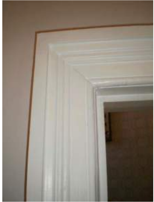
Ground floor rear room. Door architrave a modern restoration - No Significance, but high architectural merit.
