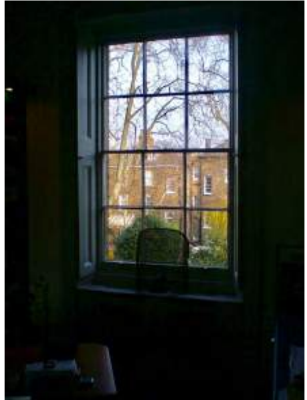
First floor rear room. Original window and shutters - High Significance.
