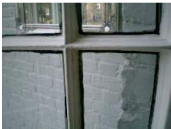
Detail of French door's glazing bars. High Significance.
