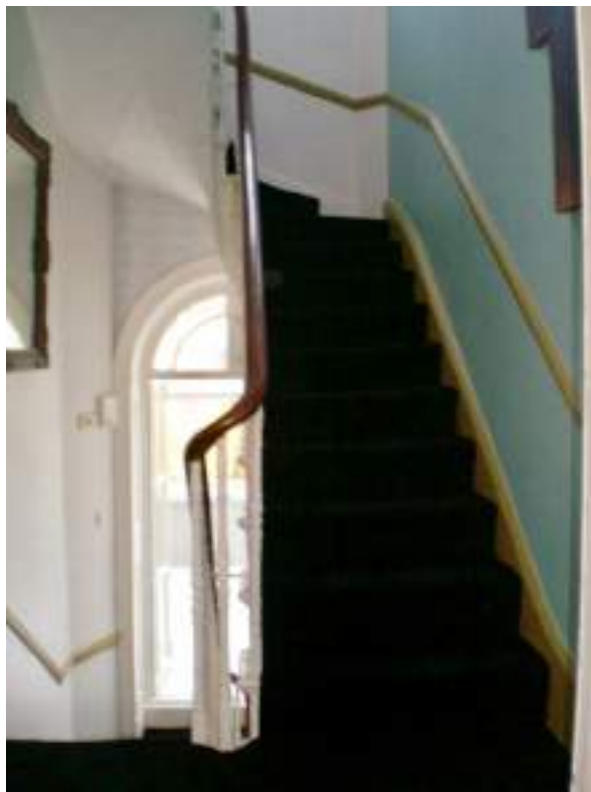
First flight from first to second floors. Original feature - High Significance.
