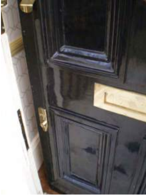
Front door detail. Flat recessed panels with bolection mouldings. High Significance.
