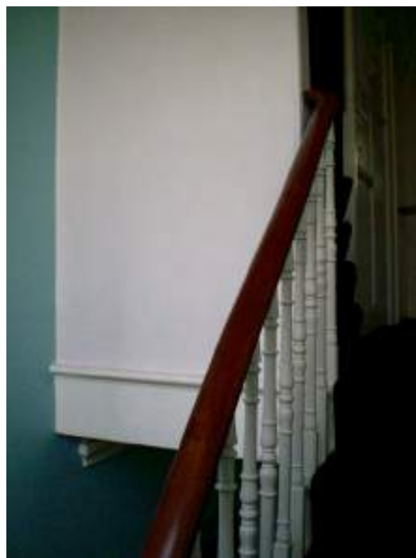
Handrail and bannisters terminating at second floor level. Original feature - High Significance.
