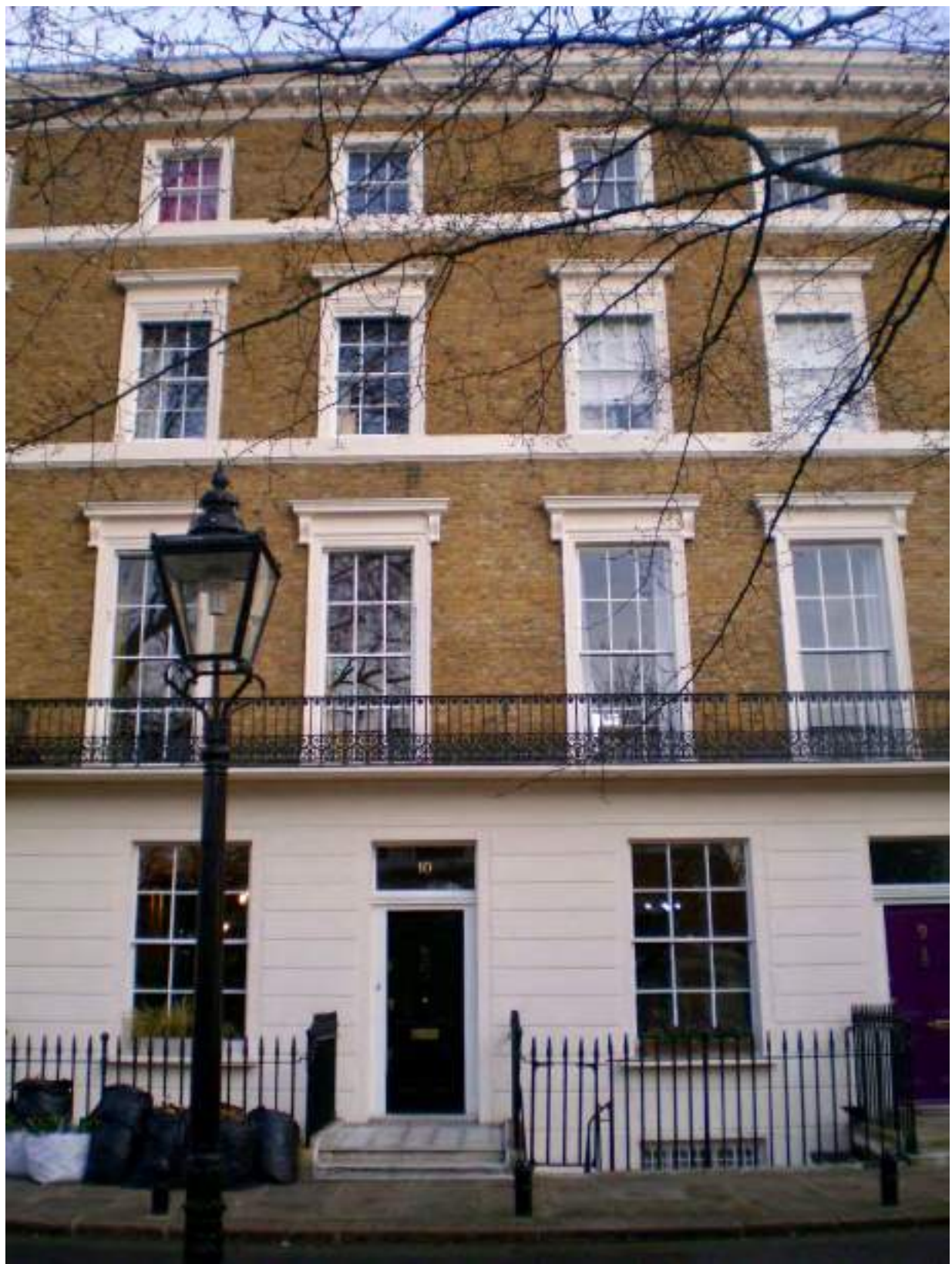
No. 10 The front Elevation. Overall - High Significance
