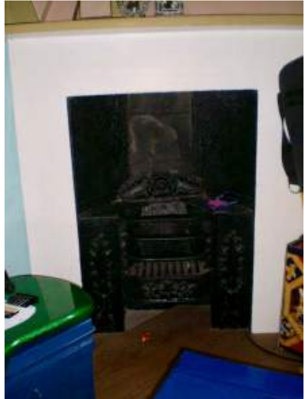
Third floor rear north bedroom. Original corner fireplace with hob grate - High Significance.
