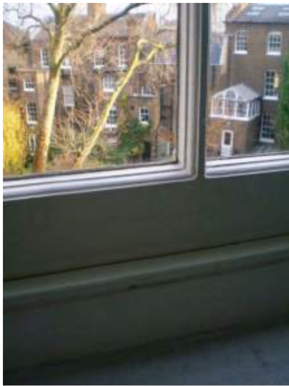
Second mezzanine level stair window. Modern replacement. Sash frame and glazing bar ovolo moulding does not match originals- No Significance. - Low architectural merit.
