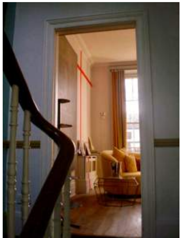
The first floor landing and swept continuous handrail. Original feature - High Significance
