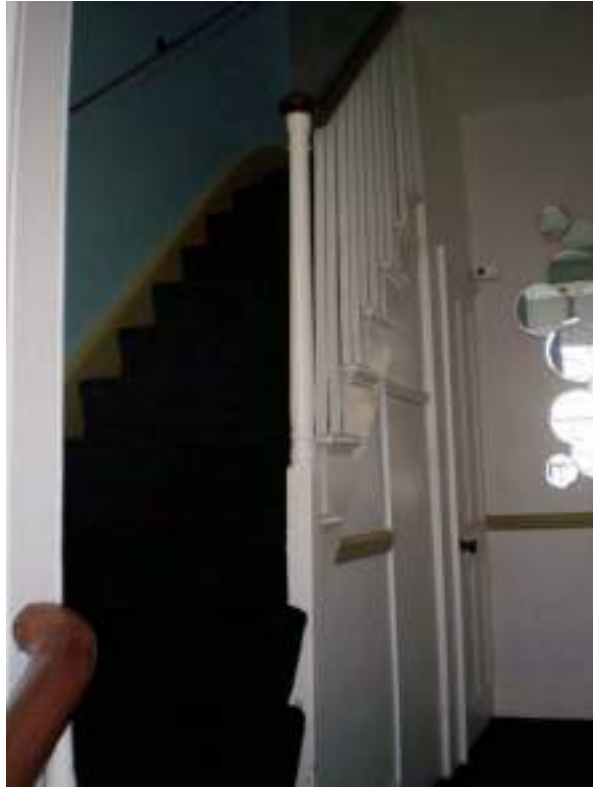
The Secondary winder stairs to third floor. Original feature - High Significance
