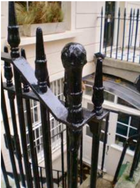
Foliated pointed finials to common rails and ball tipped foliated finial to queen post - High Significance.
