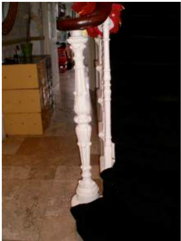
Ground floor stairs, cast iron ornate newel post. Original feature - High Significance.
