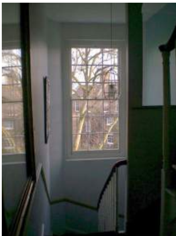
Second floor level staircase window. Enlarged by lowering Cill - No Significance. High architectural merit.
