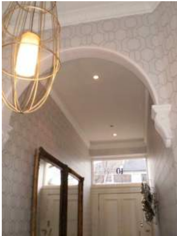
The entrance hall bracketed arch. Original feature - High Significance
