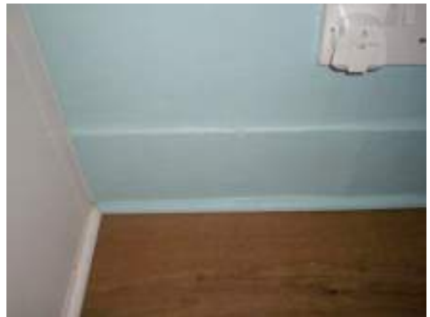
Third floor front south bedroom. Original skirting board - Low Significance.
