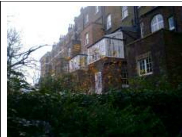
The rear of the houses to the south side. Conservatories on top of the rear wings.
