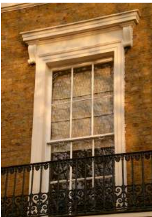
Detail of First Floor Window with bracketed cornice - High Significance
