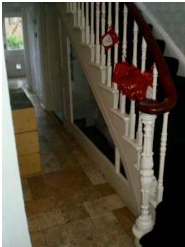
Ground floor stair. Original feature - High Significance. Panelling to underside removed and replaced with glass - Harmful modern alteration.
