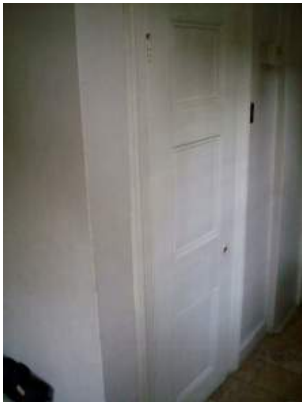
Ground floor rear wing. WC. Original door - Medium Significance.
