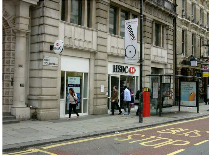
PHOTOGRAPH OF FRONT ELEVATION
