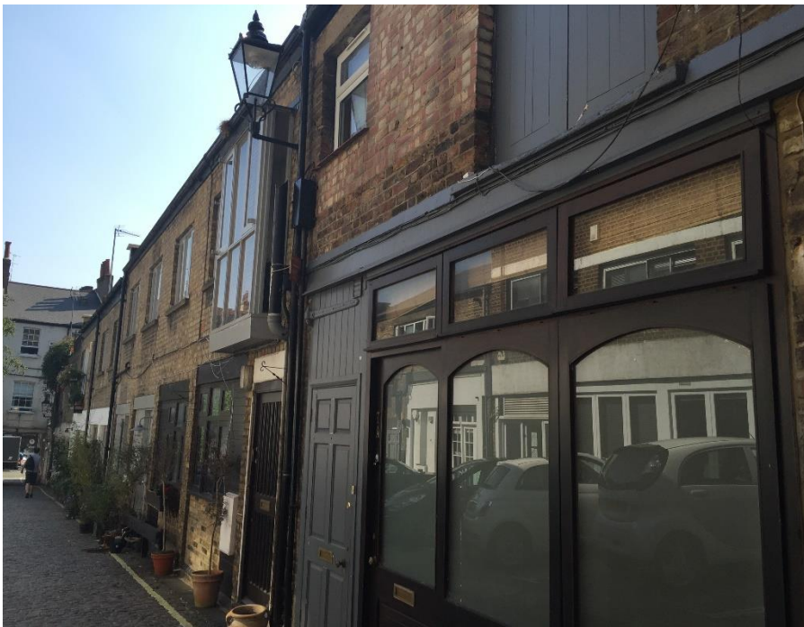
South side of the Mews – Residential
