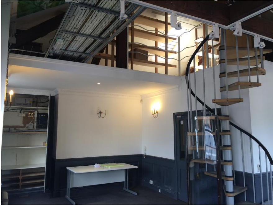
Figure 9: Tack Room: first floor: north bay. The partitions and mezzanine floor are modern and to be removed.
