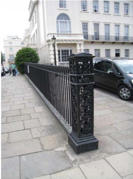
Photo no. 12 Box standard Listed Railings RL14 (part of EH list entry no. 1244298)
