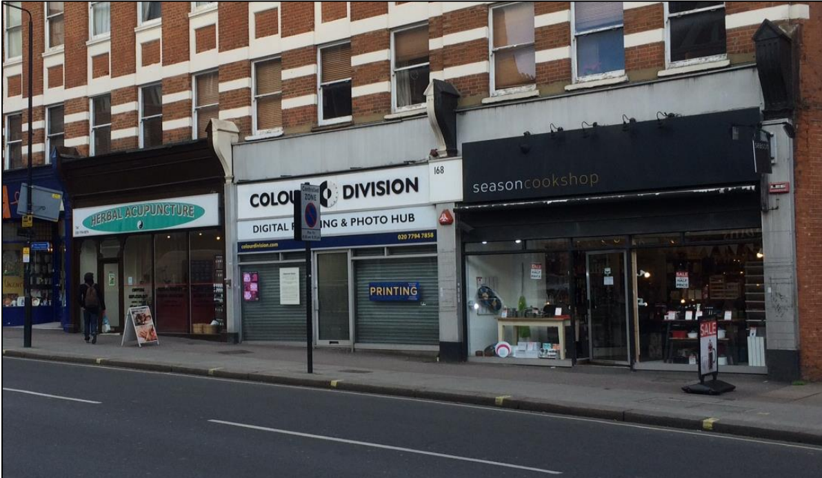
Photograph of existing vacant unit at no.168 West End Lane (central) and adjoining units
