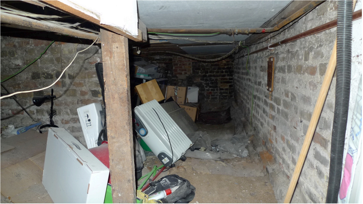
Fig. 5 Basement looking towards front elevation
